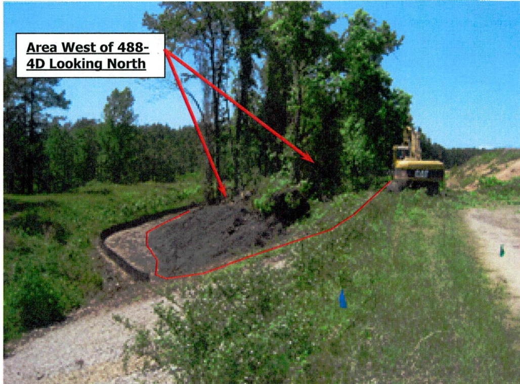
Photo 20. Start of Clearing and Grubbing 488-4D West End
