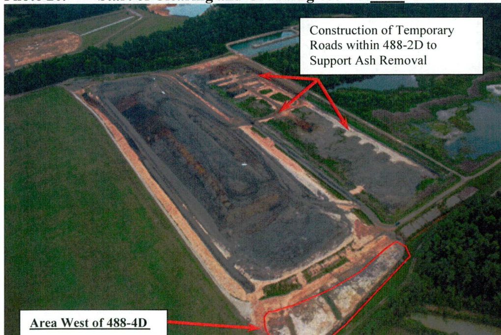
Photo 24. Construction of Temporary Roads within 488-2D
