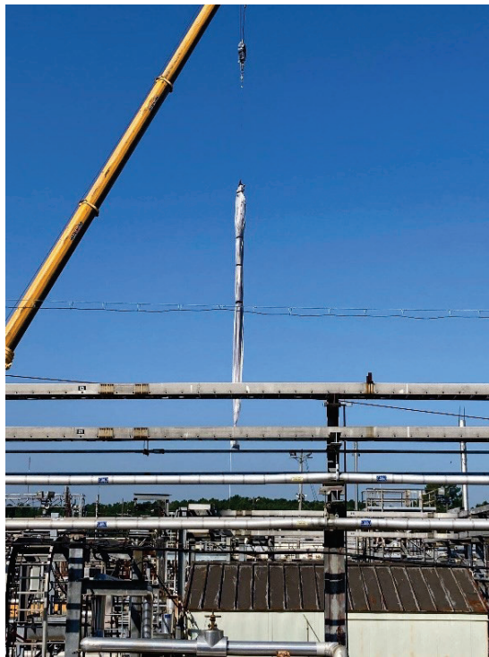
Figure 1: Tank 3F Caisson D&R
