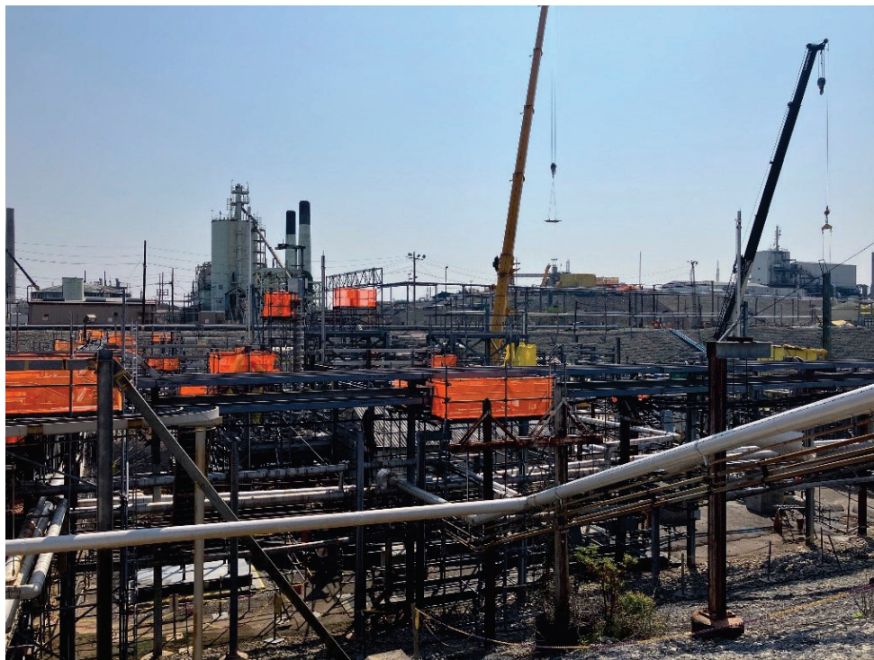
Figure 5: Tank 10 STP Replacement
