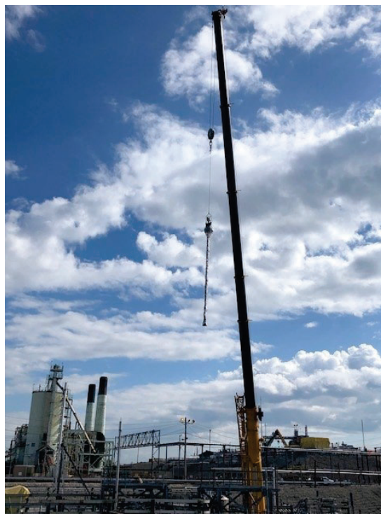
Figure 3: Tank 9H Riser 4 LVMJ Removal
