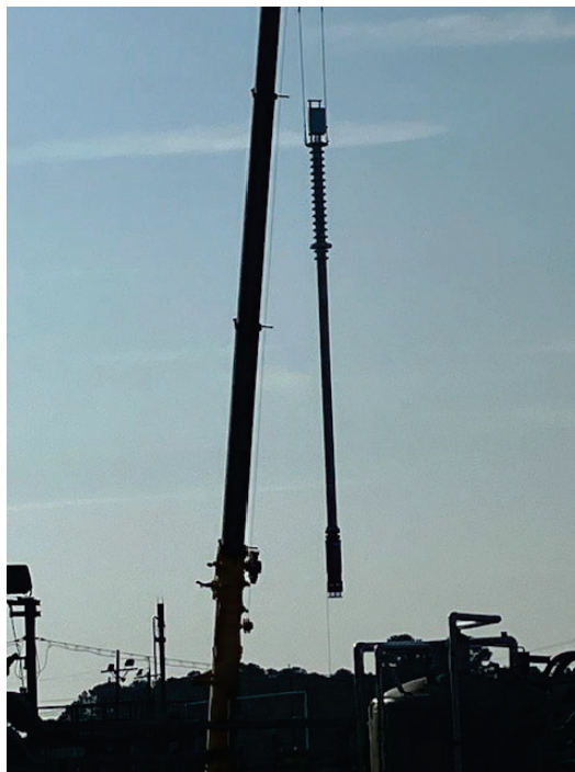
Figure 2 – Tank 3F Riser 6 CSMP Installation
