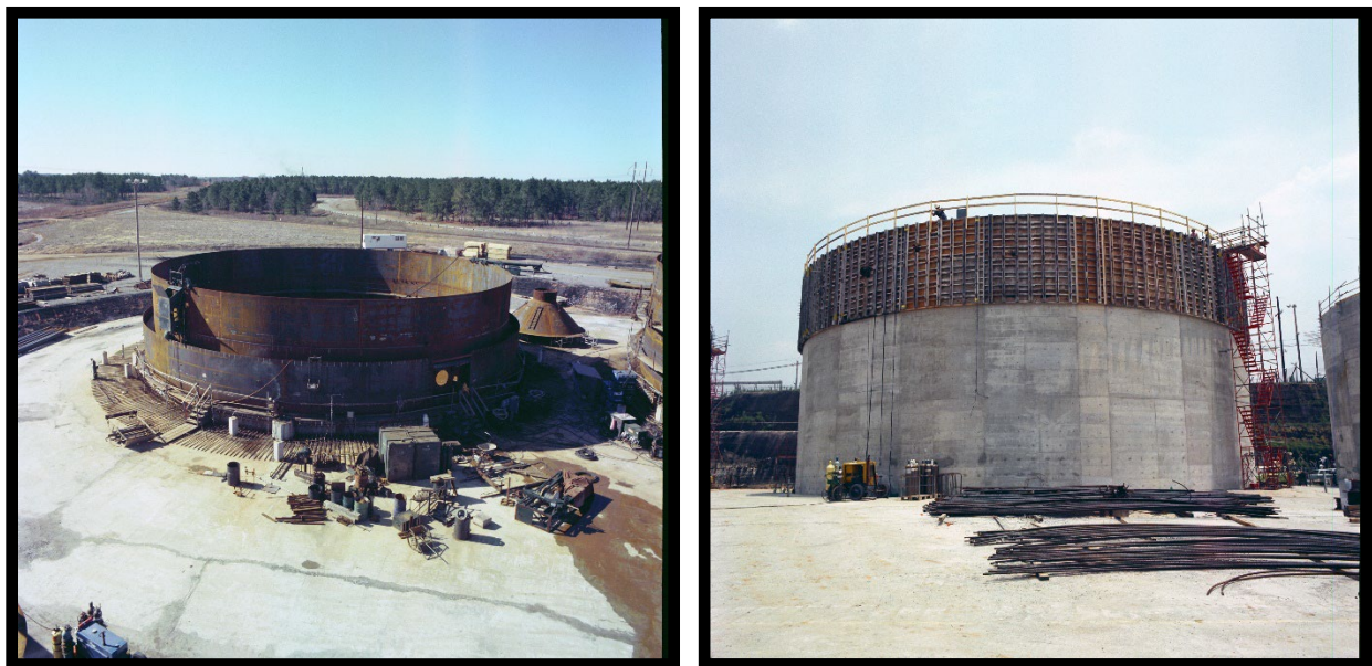
Figure 3.4-1: Typical Construction of Type III/IIIA Tanks
