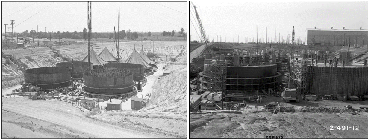
Figure 3.1-1: Construction of the Type I Tanks in FTF
