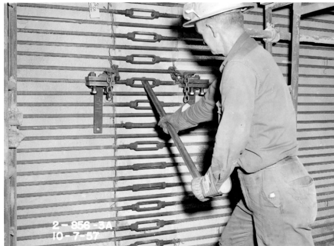
Figure 3.3-2: Steel Bands and Turnbuckles on the Type IV Tank Walls
