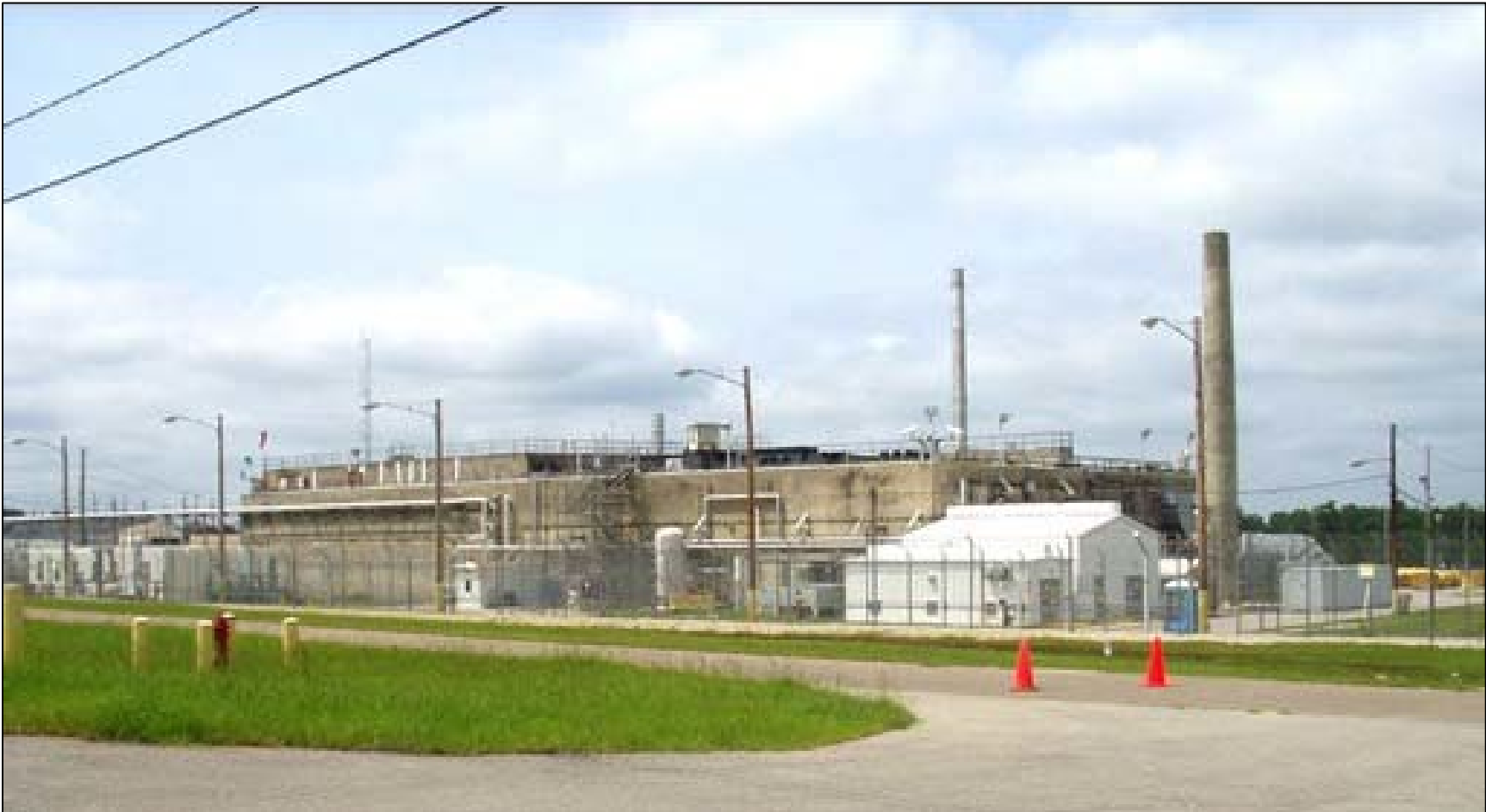
Figure 3. Historical Photograph of Building 235-F (Prior to 293-F Stack Reduction)
