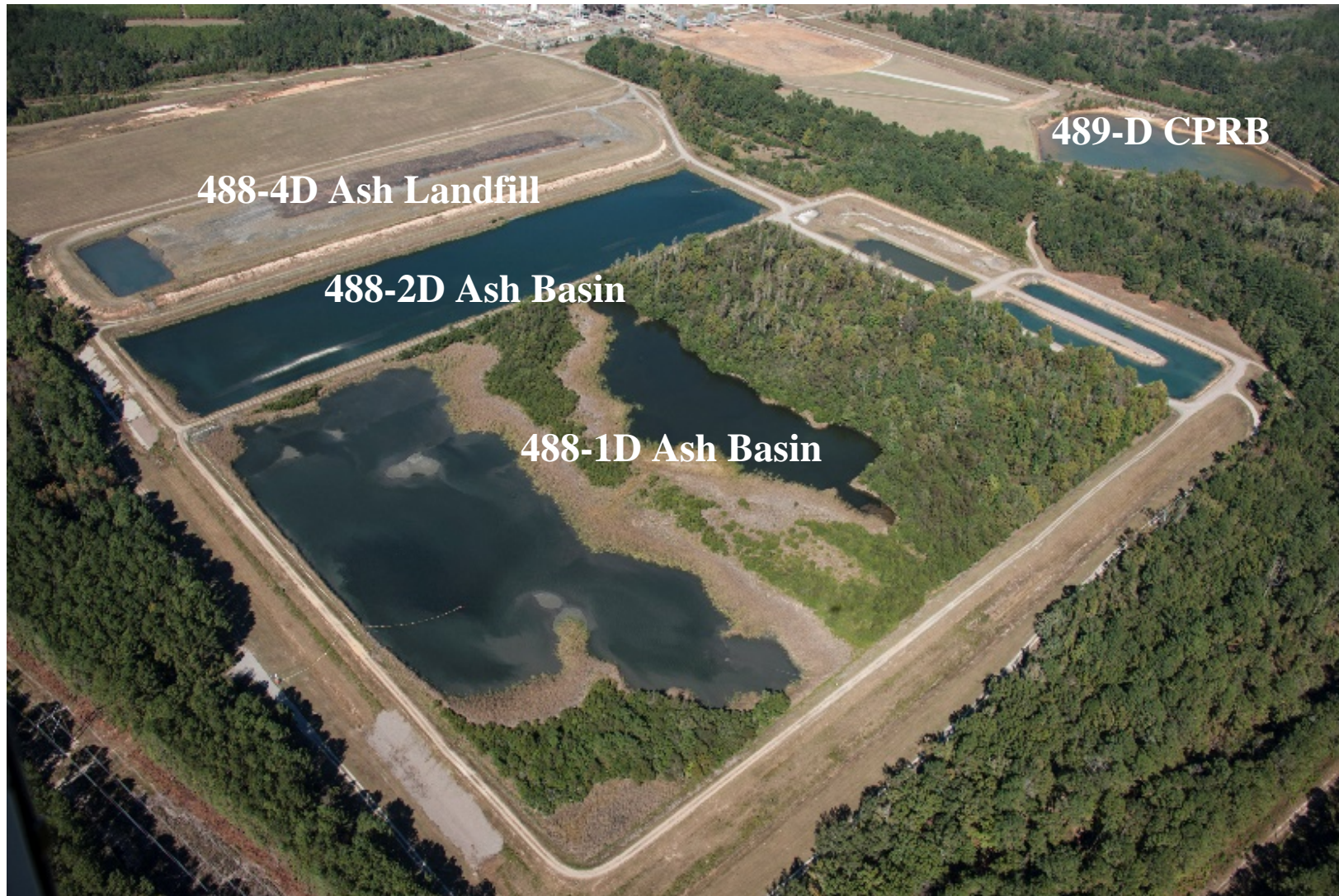
Figure 7. D-Area Project in October 2013 (Before Project Initiation)
