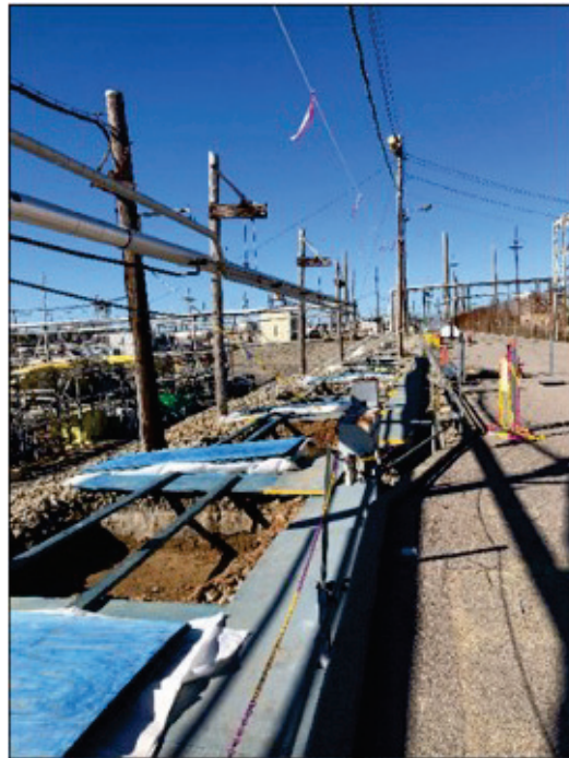
Figure 3: Pier Excavations for Chromate Water Reroute
