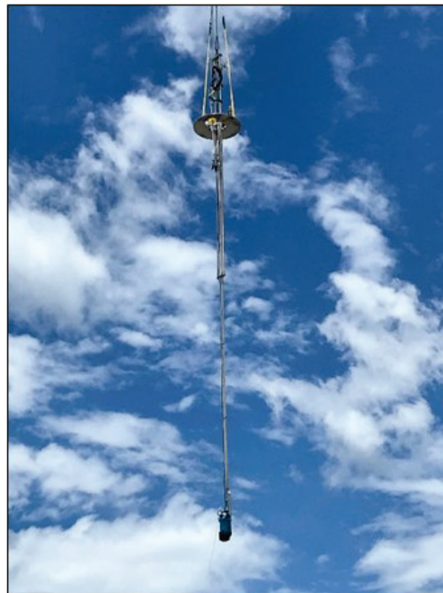
Figure 12: Tank 44F Replacement STP
