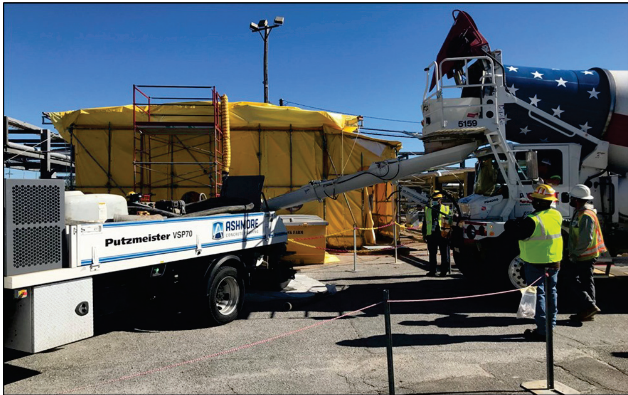
Figure 15: FDB-5 Grout Delivery
