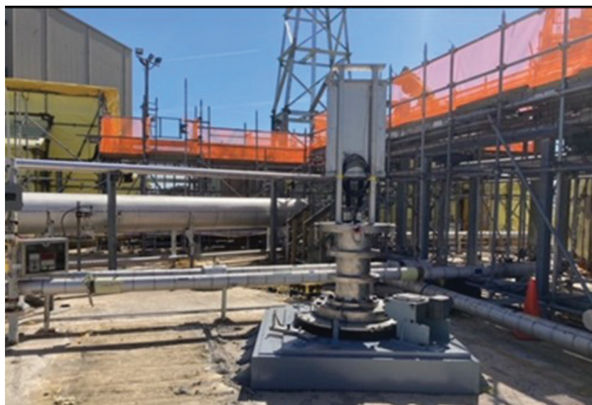
Figure 9: Tank 35H CSMP Installation at Riser B8
