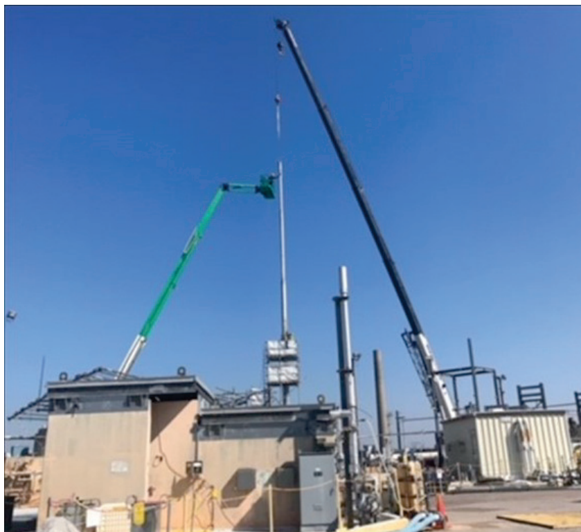
Figure 10: Tank 39H Stack Extension
