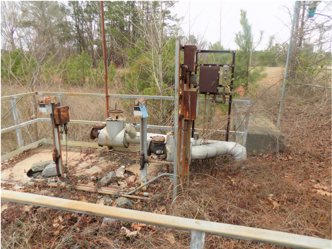
Figure 15. 483-6D Surge Basin Remnants
