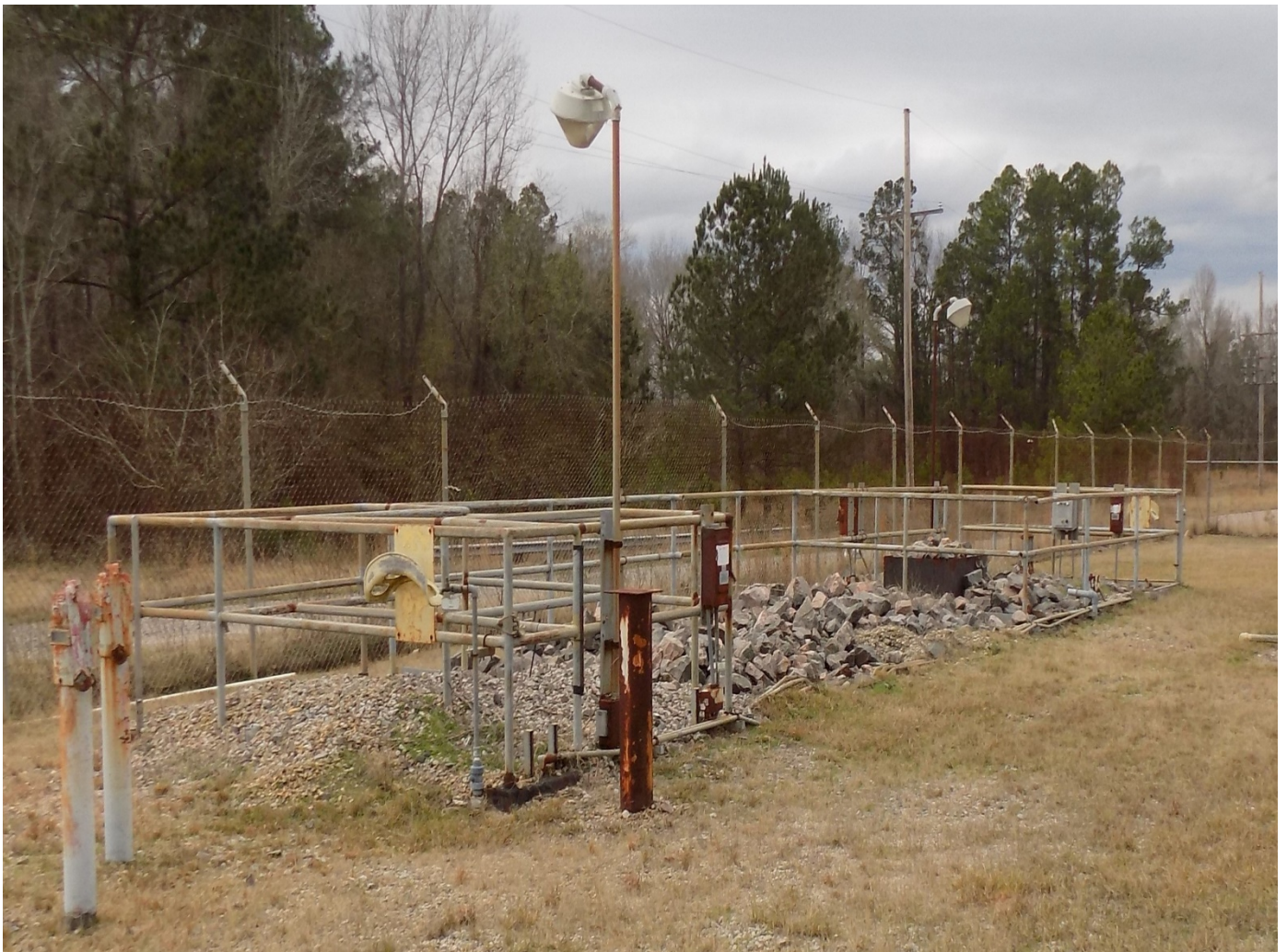
Figure 9. Building 607-15D, Sanitary Waste Treatment Plant
