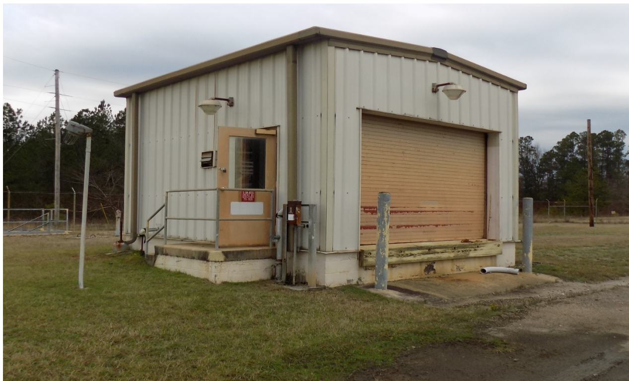
Figure 4. Building 607-14D, Chemical Feed Building
