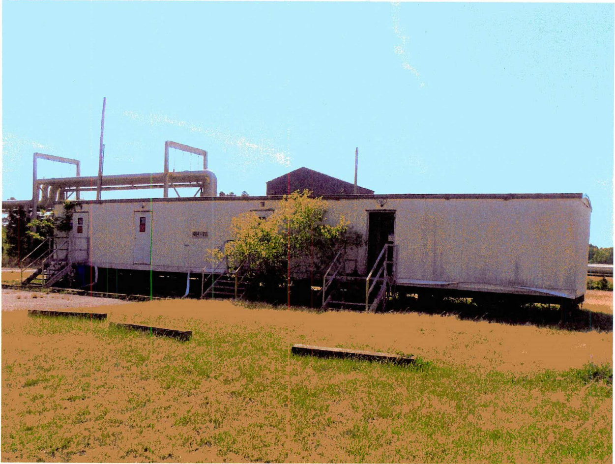
Figure A-3. Building 484-2D Before
