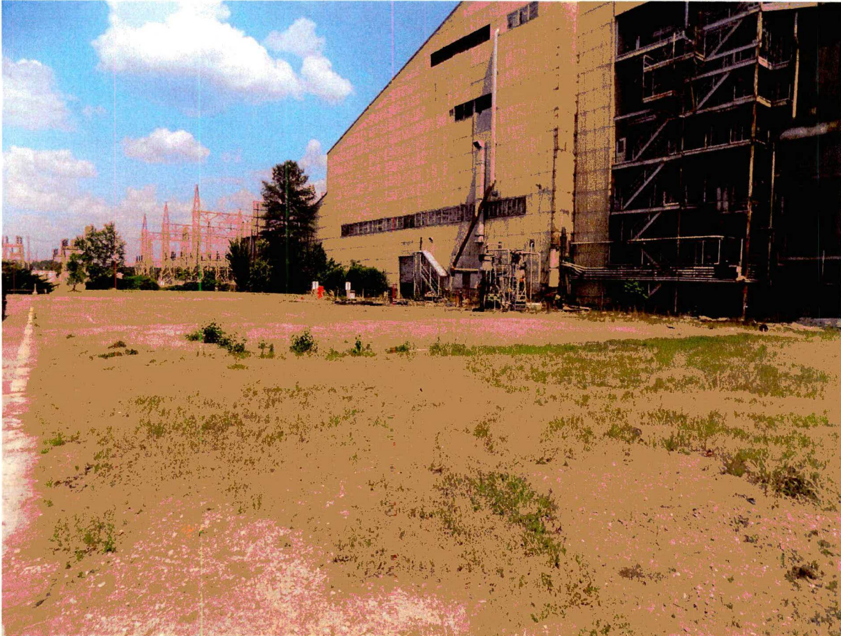
Figure A-2. Building 484-1D After
