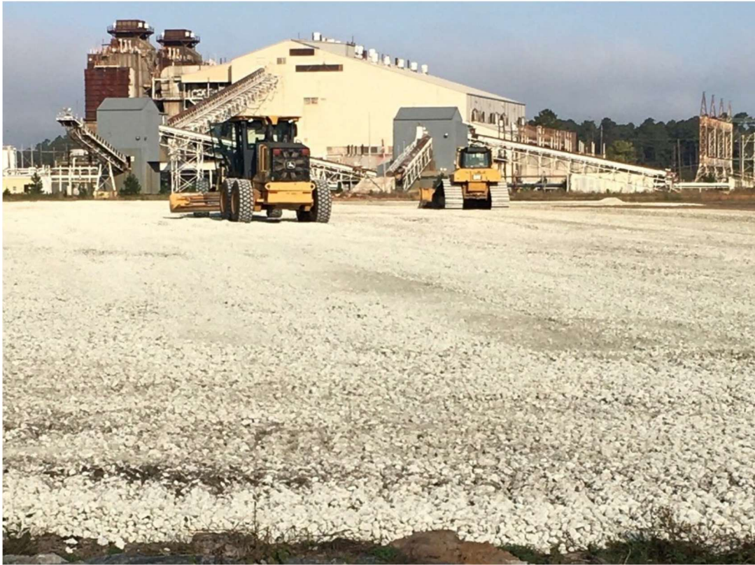
Photo 6. Placement of Limestone Gravel Stabilization
