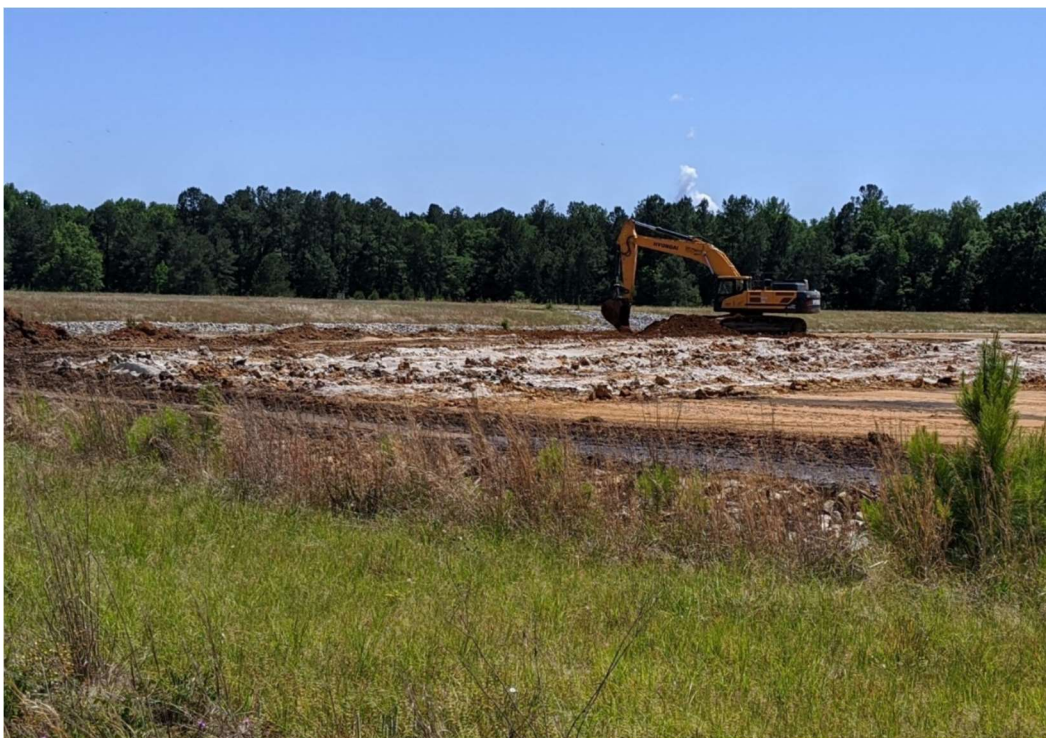
Photo 4. Excavator Removing Four Feet of Soil and Amendment
