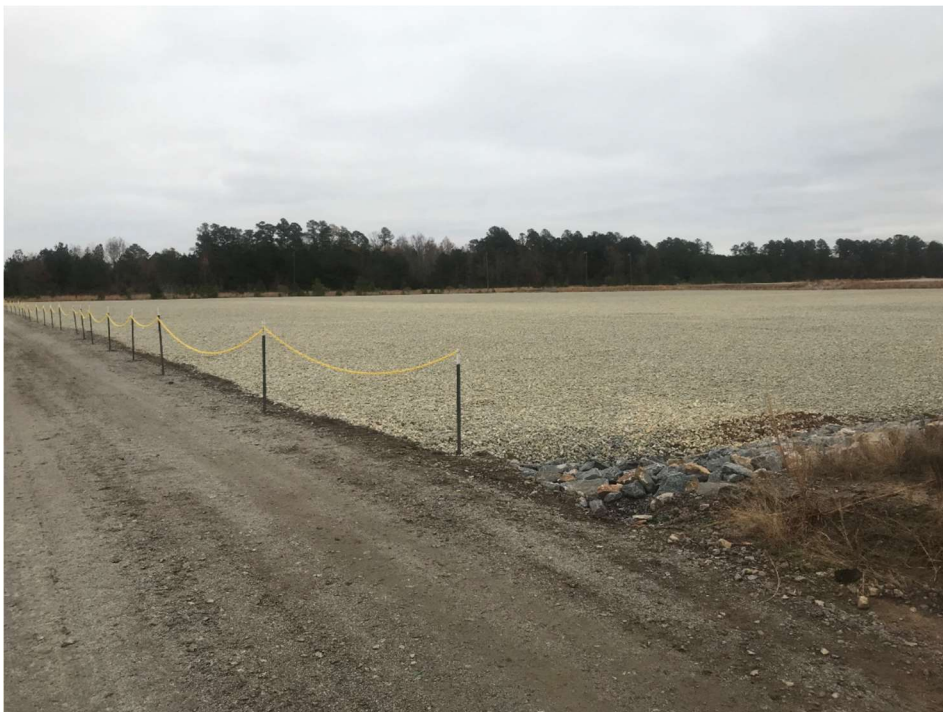
Photo 9. Plastic Chain and Post Barricade (Used to discourage vehicle access to limestone gravel cover.)
