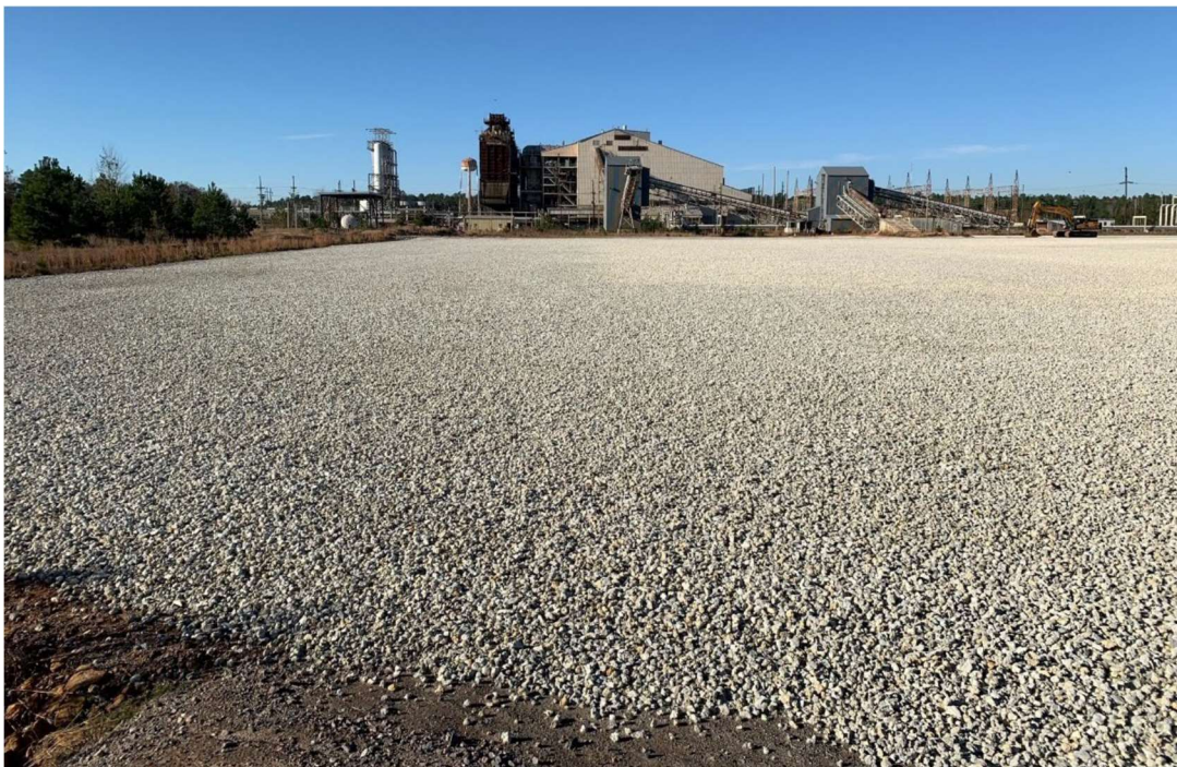
Photo 7. Finished Limestone Gravel Cover
