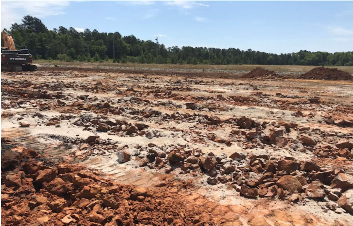
Photo 3. Amendment Spread over Decompressed Soils
