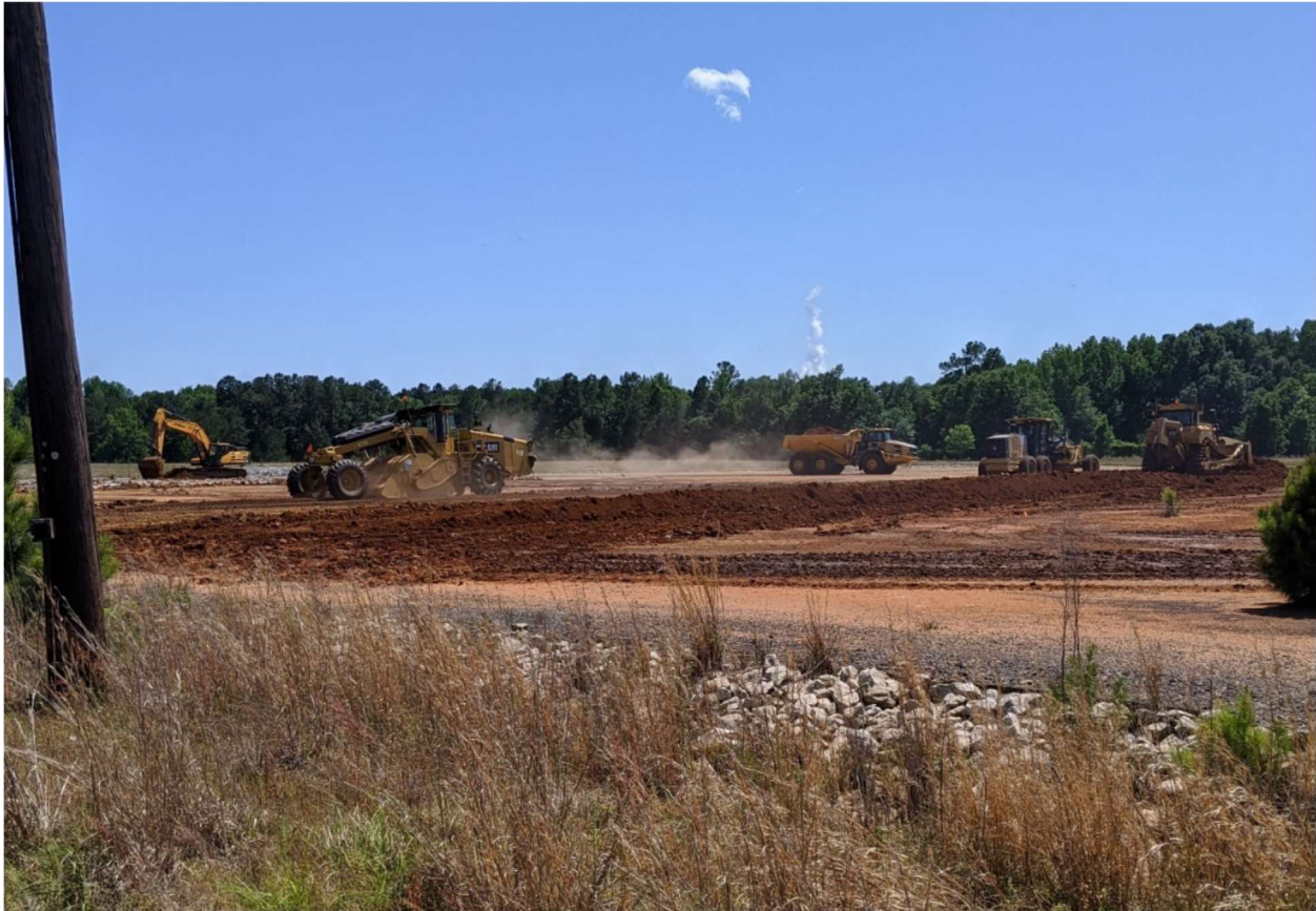
Photo 5. Equipment Types Used (From left to right: excavator, processor, dump truck, grader, and bulldozer work to mix amendment)
