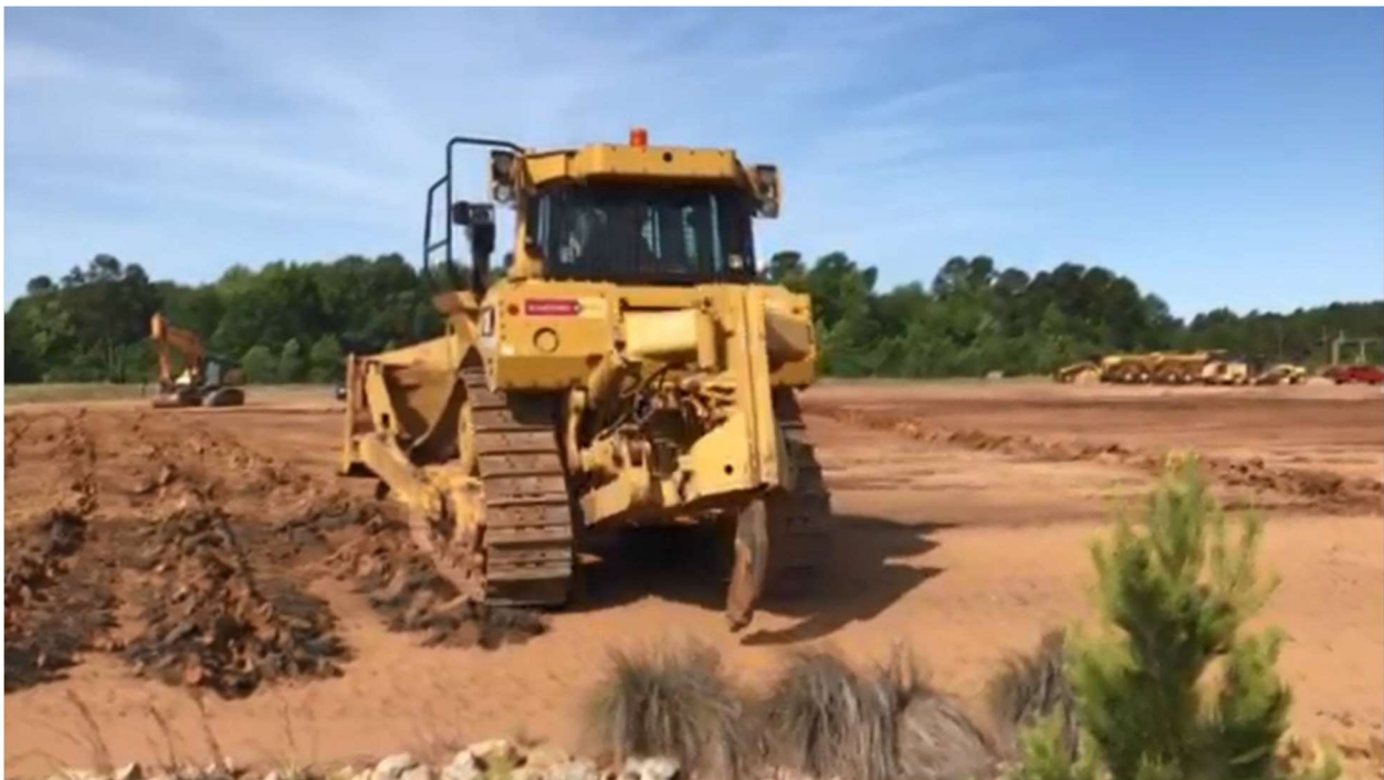
Photo 2. Bulldozer with Ripper Attachment Decompacting Coal Yard Soils
