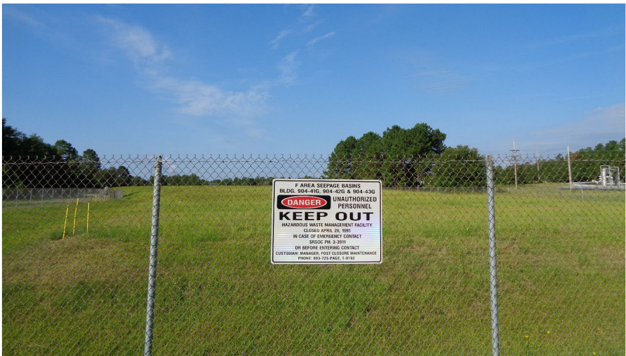
Figure E-3. Current On-Unit Photographs of the Cover System of the FHWMF OU (2020)
