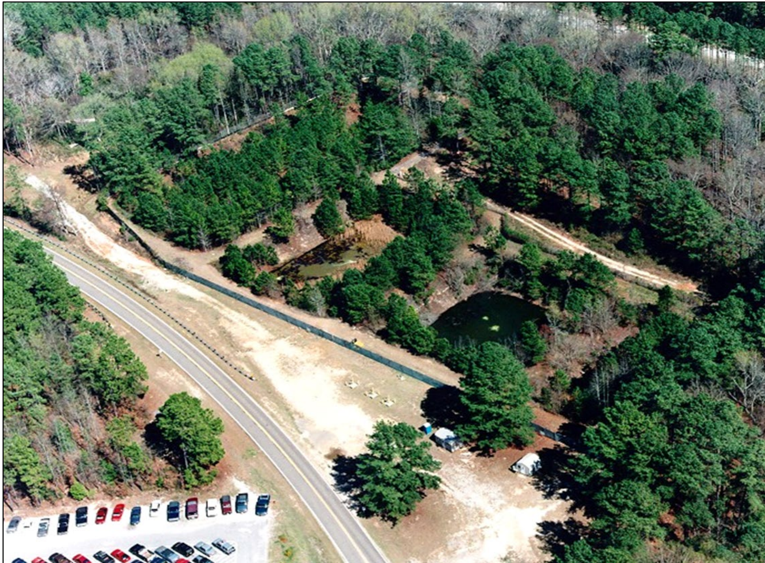
Figure L-3. Photo of SRLSB OU Before Remediation Activities
