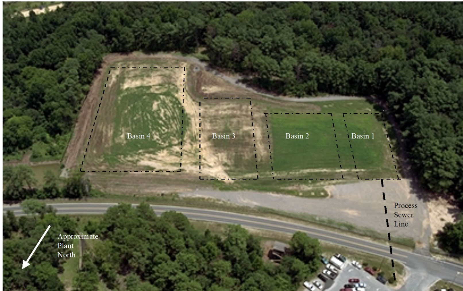
Figure L-2. Layout of the SRLSB OU (904-53G, 904-53G, 904-54G, and 904-55G) after Construction Completion (2001)
