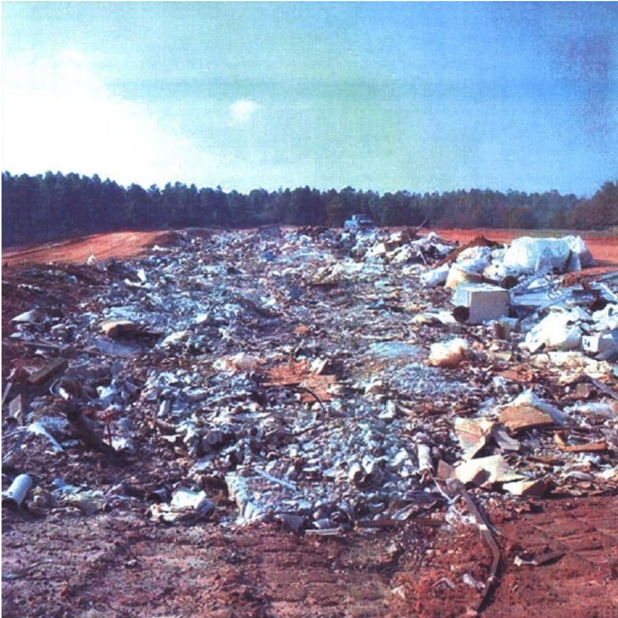
Figure C-3. Photo of CSBRP OU Before Remediation Activities (1985)
