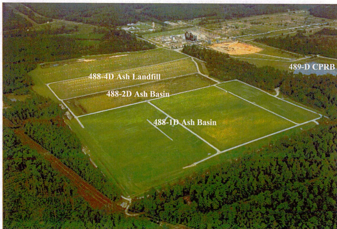
Figure 5. D-Area Project in October 2018 (After Project Completion)
