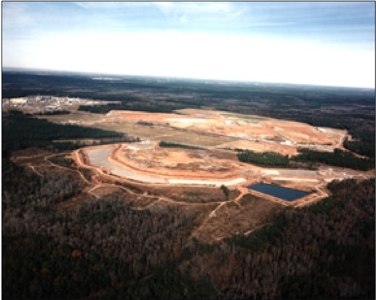
Figure I-2. H-Area HWMF Basins Prior to Closure (1989)
