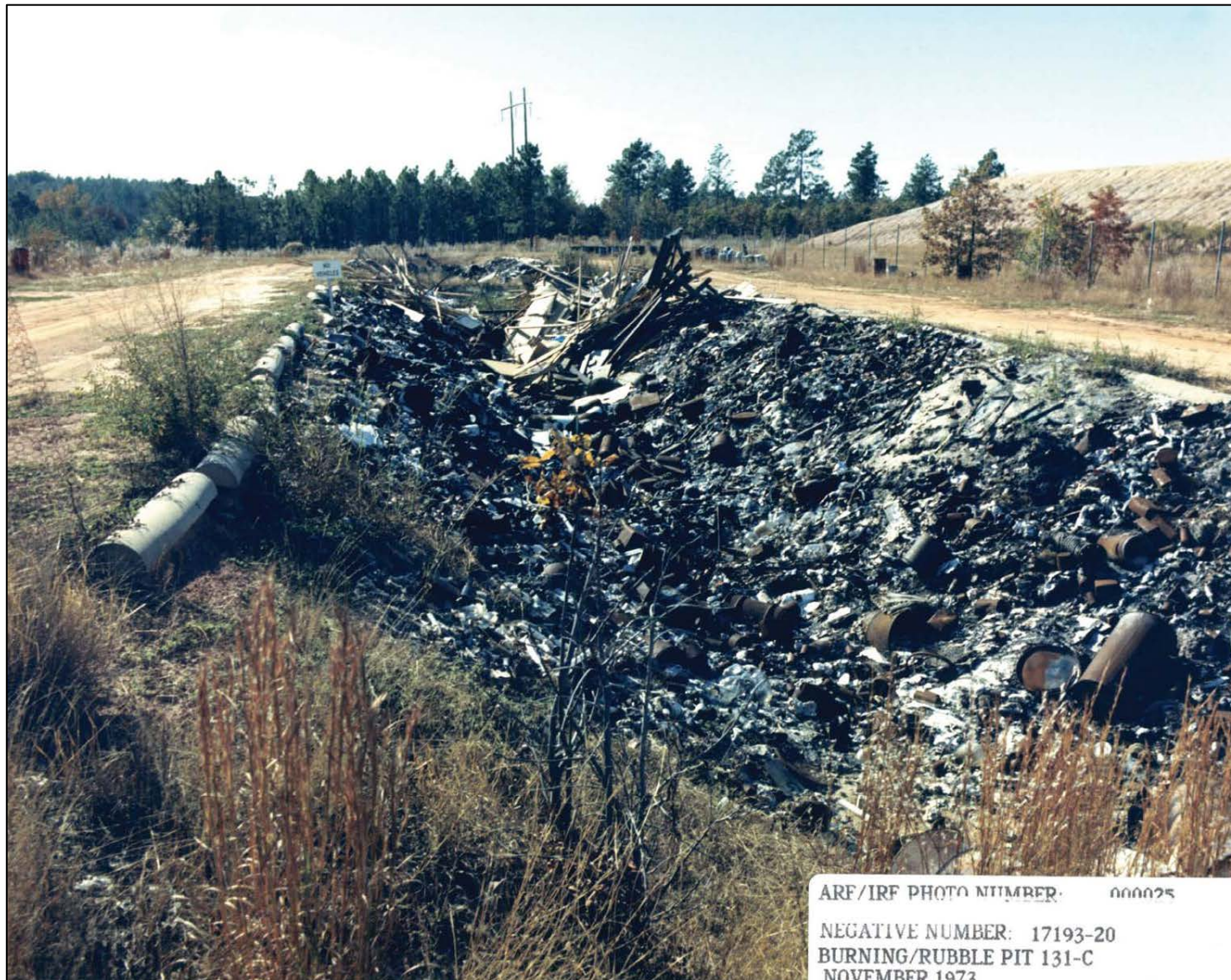
Figure F-4. Photo of CBRP Before Remediation Activities (1973)
