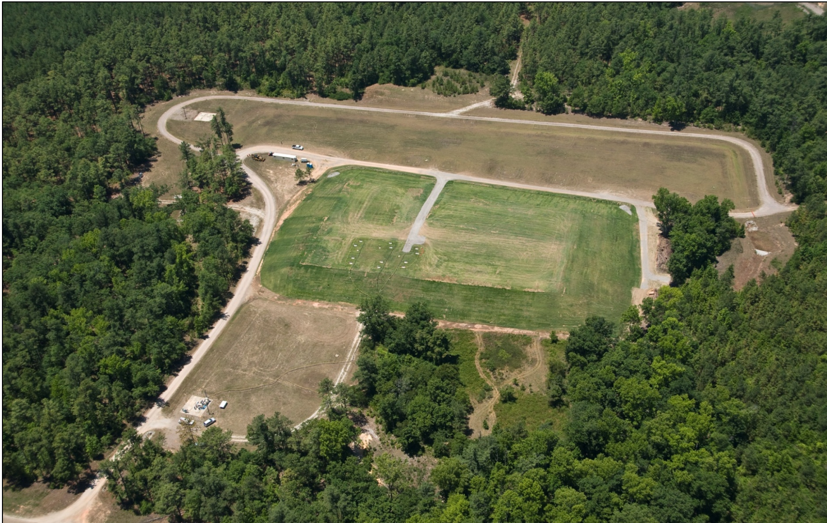
Figure C-6. A-Area Ash Pile and Underlying Trench Subunit after Final Action, with Installation of Trench Subunit SVE System (2008)
