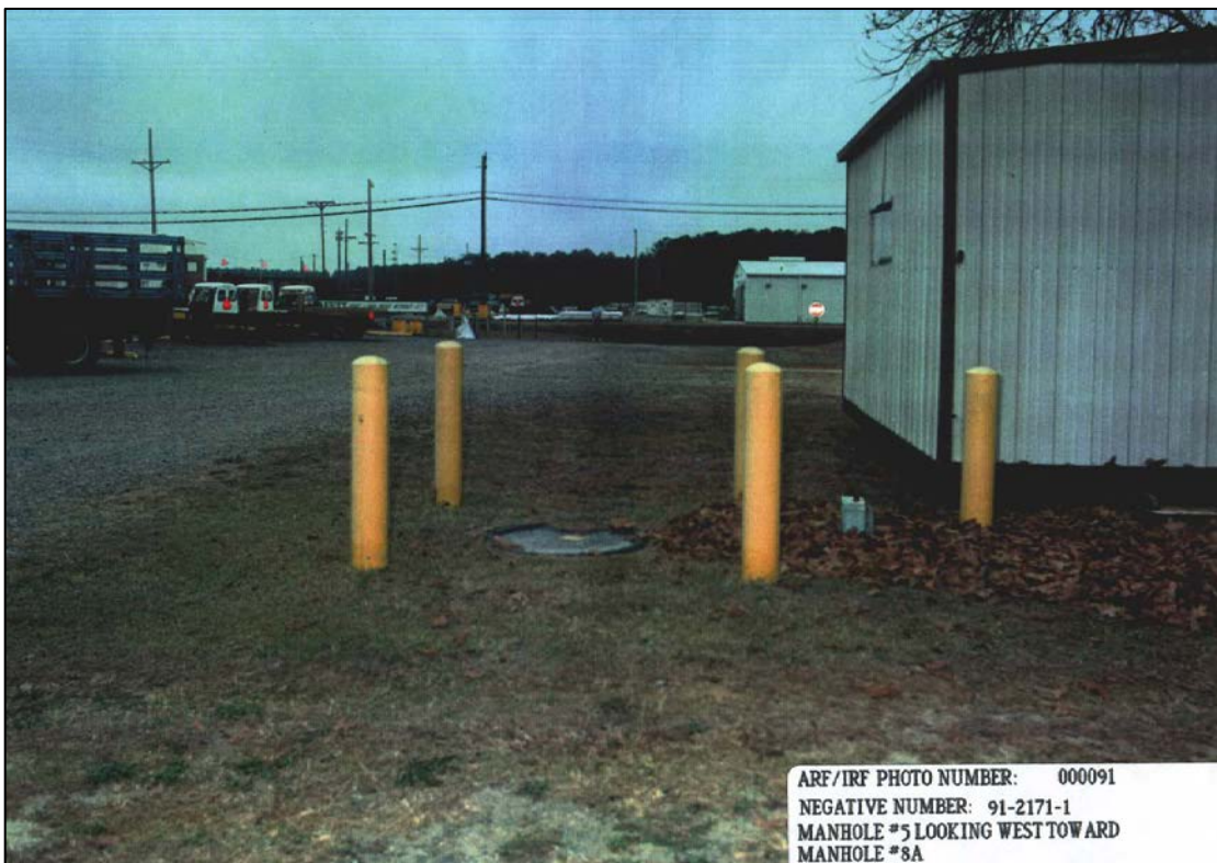
Figure K-3. Photos of MIPSL OU Before Remediation Activities (1991)
