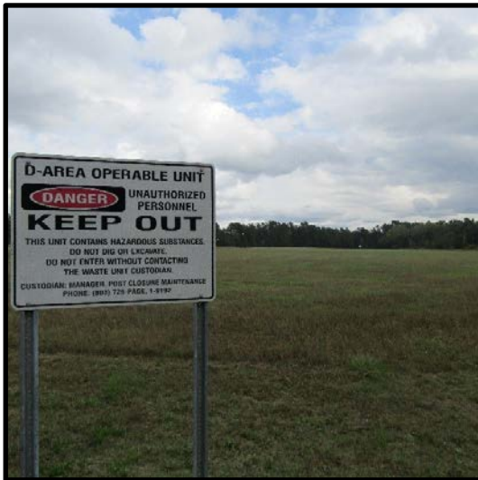
Coal Pile Runoff Basin
