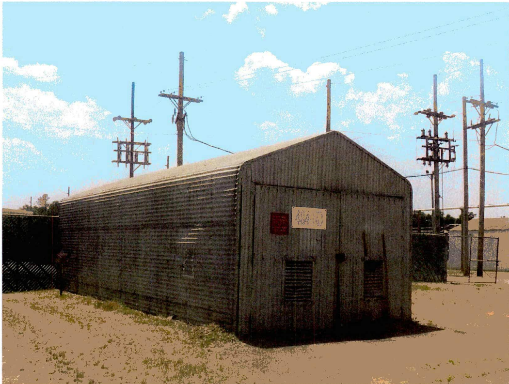
Figure 3: Building 484-5D, Storage Building Photo
