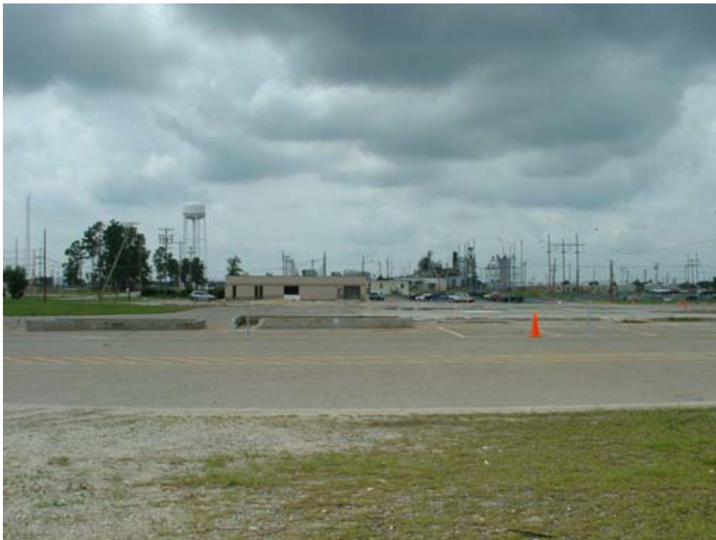
Figure 9. Building 716-A Remnant Slab, After Decommissioning
