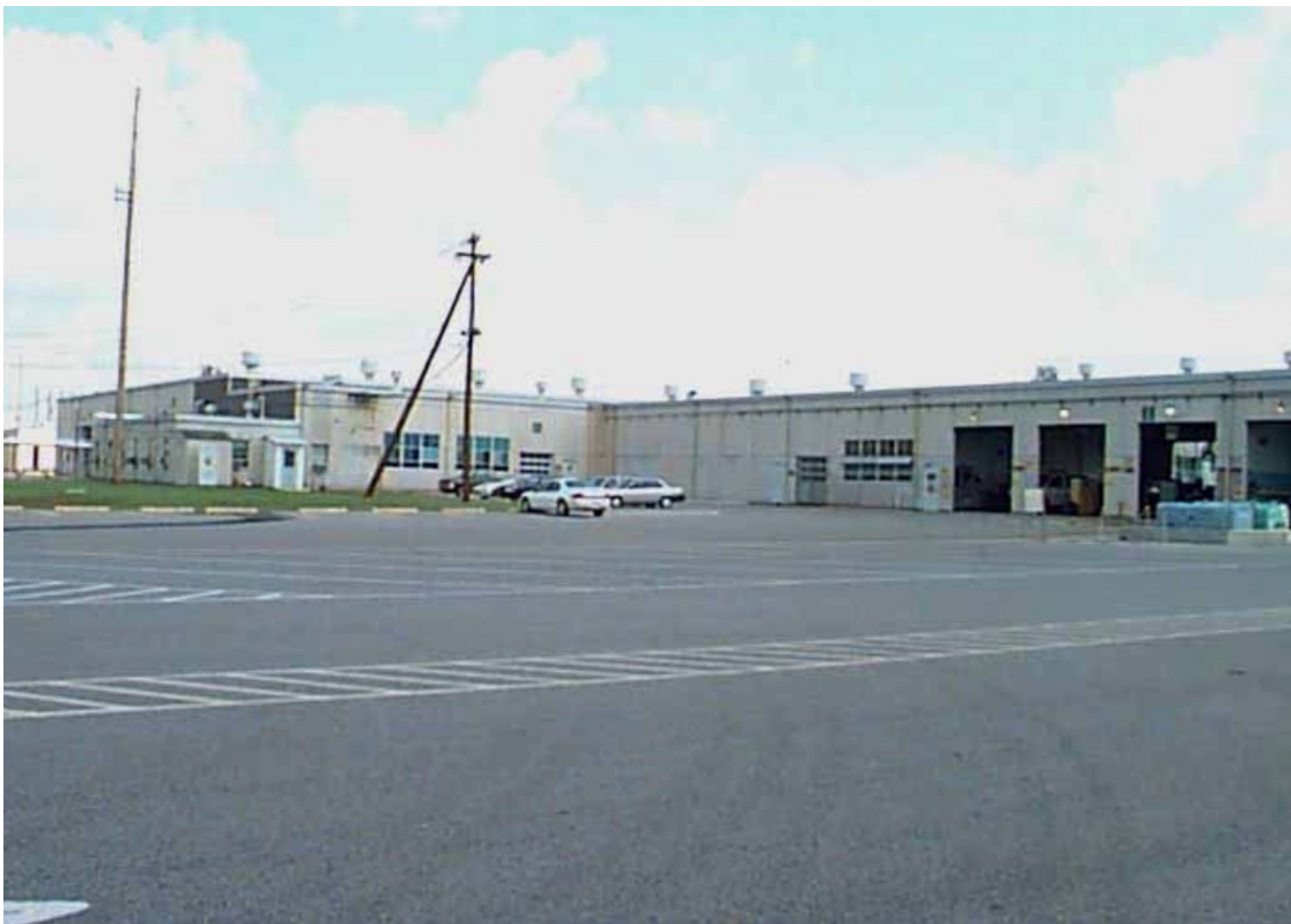
Figure 8. Building 716-A, Before Decommissioning
