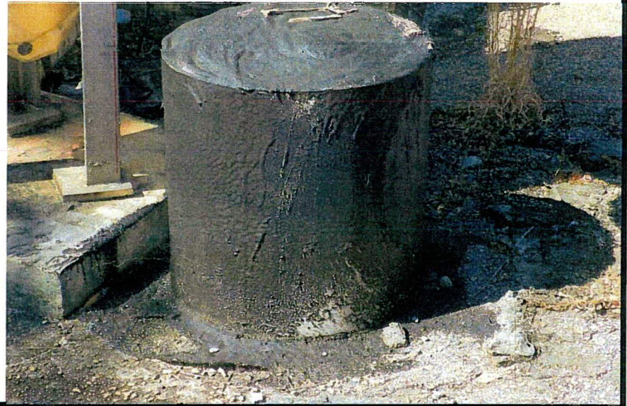
Tank 20, Ventilation Riser
