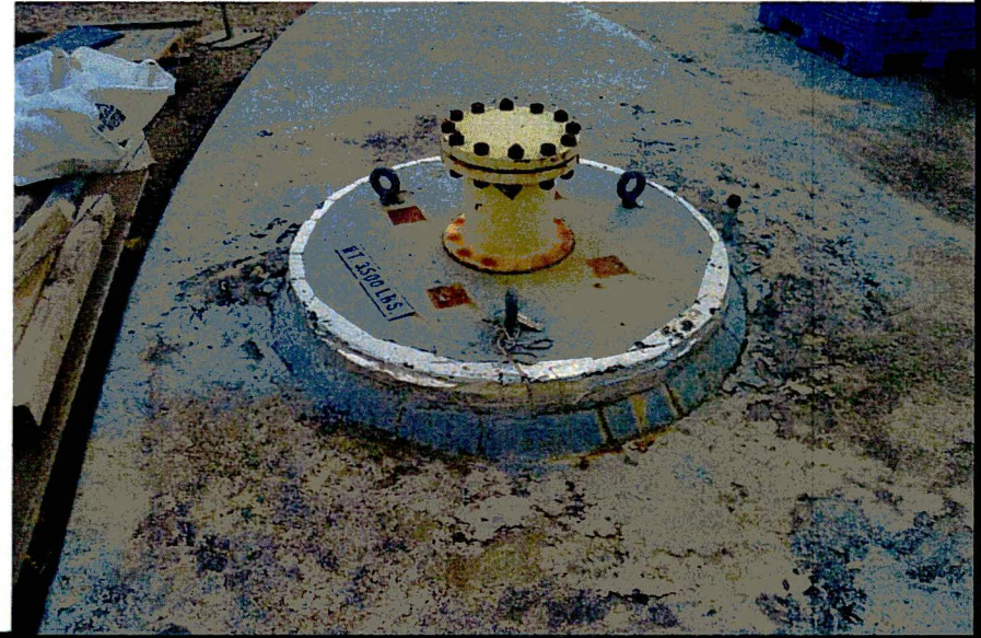
Tank 16, North Annulus Riser
