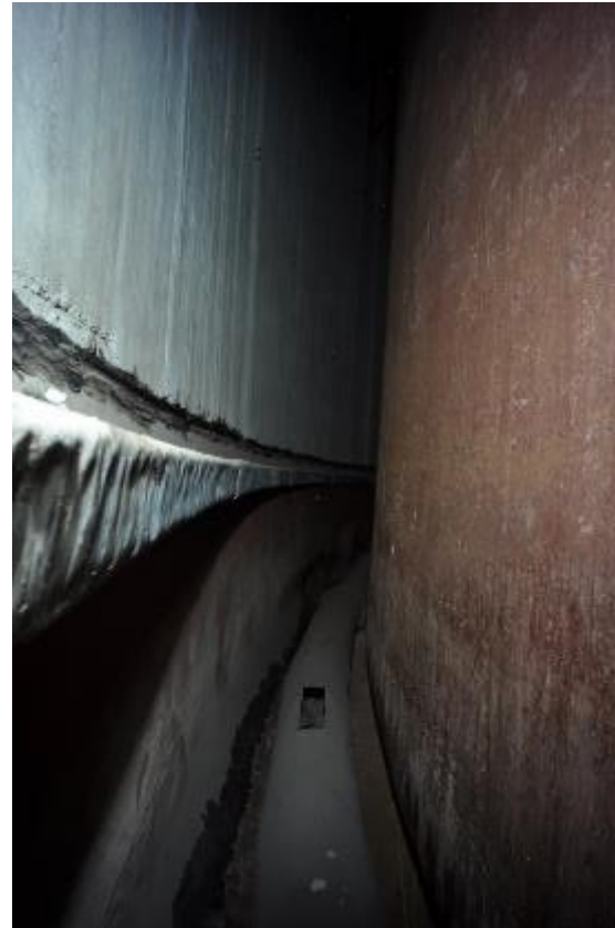
North Riser Facing East
