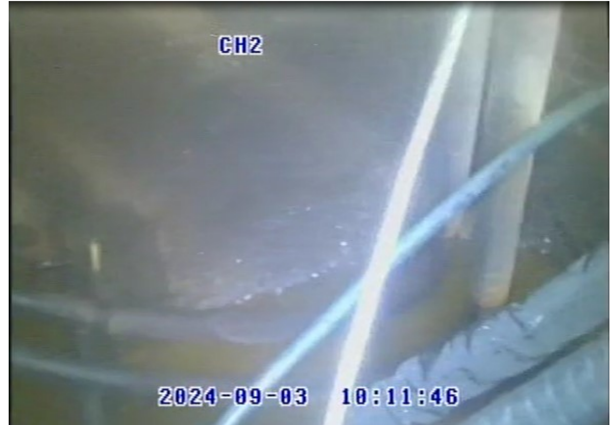
Riser 6 mound looking towards SW tank wall
