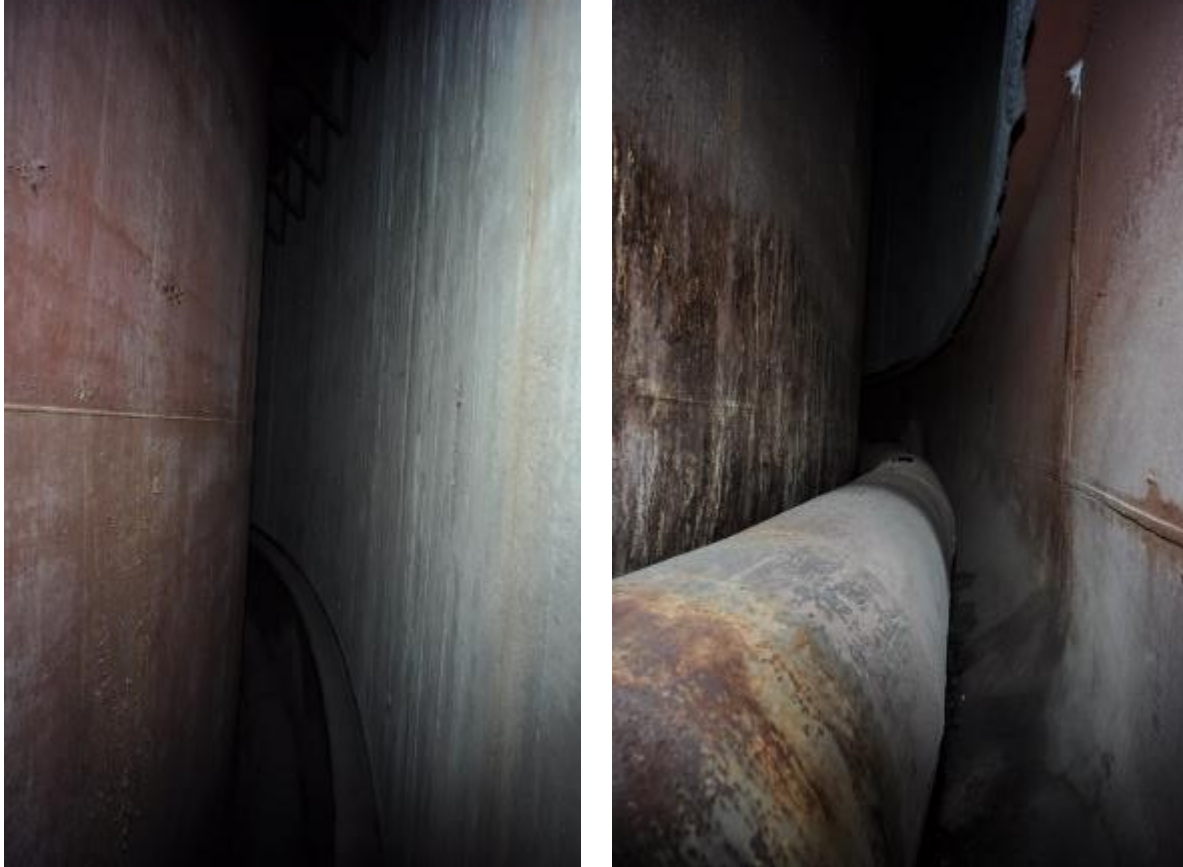
South Riser Facing East
