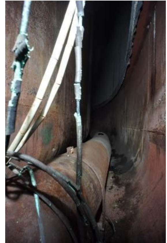
North Riser Facing West
