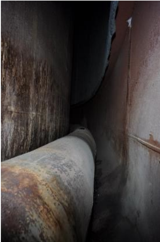
South Riser Facing East
