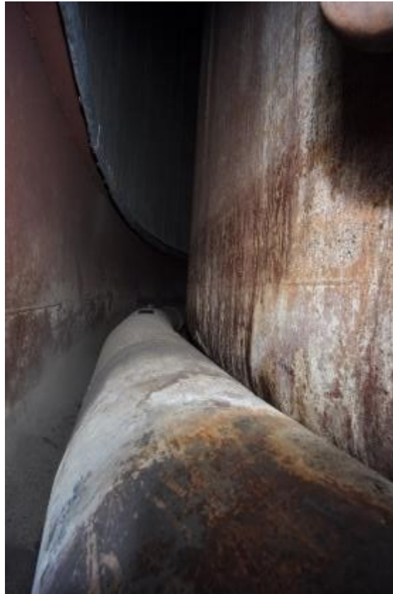
South Riser Facing West
