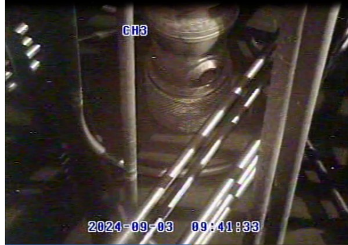
Riser 2 looking NW (Riser 3 SMP)
