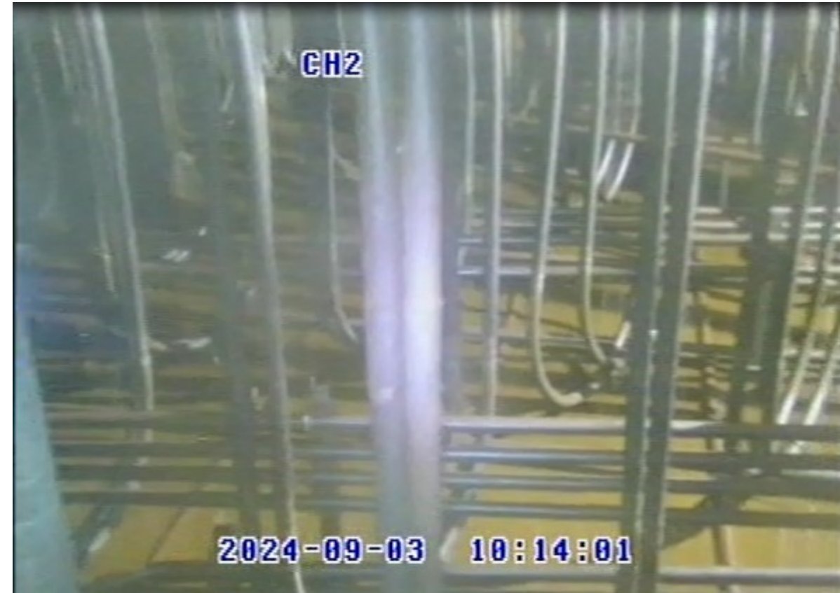
Riser 6 looking towards SW-S tank wall
