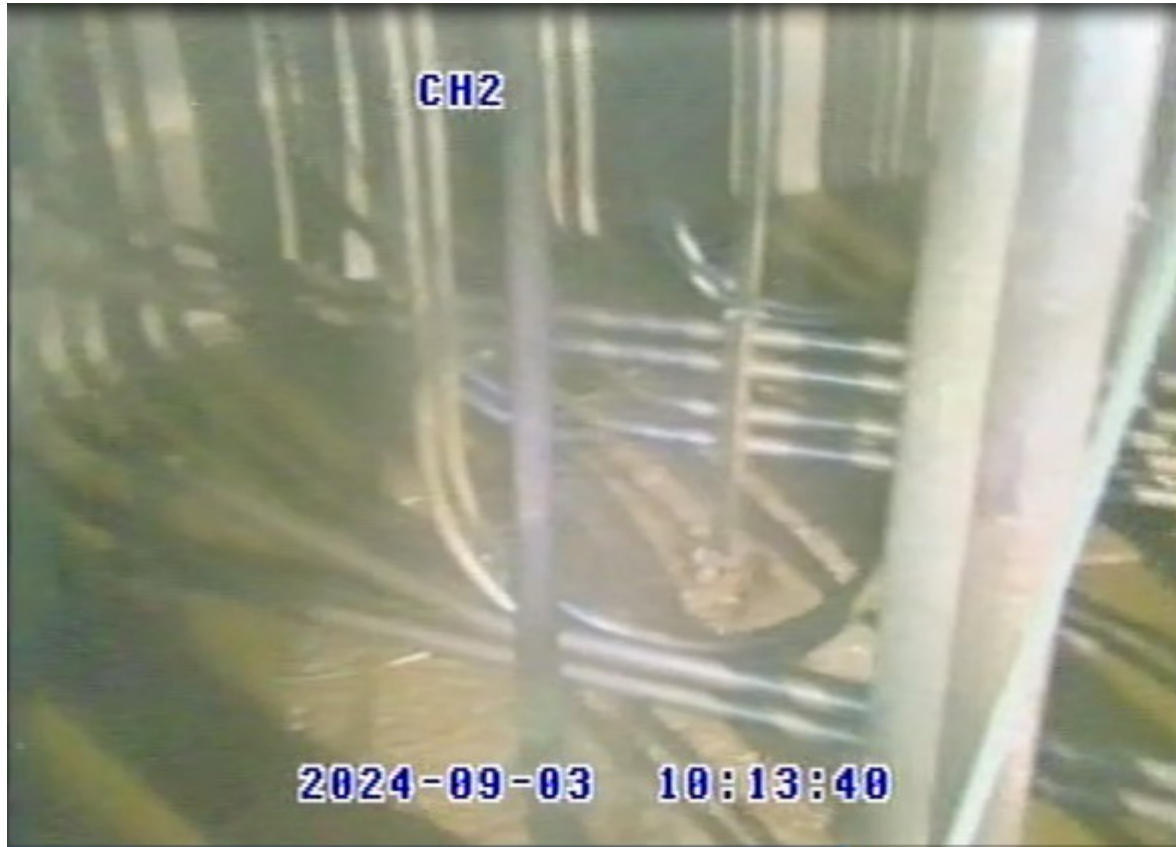
Riser 6 mound looking towards SW wall
