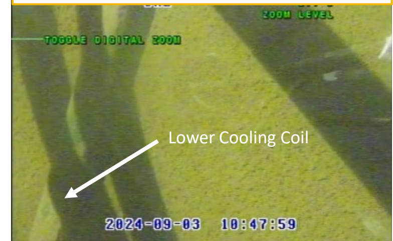
Tank Floor NE Quadrant
