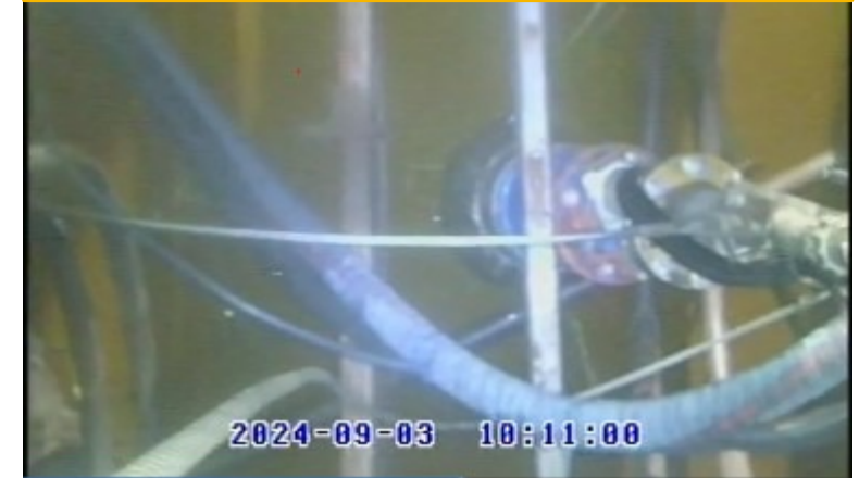
Riser 6 STP Lower Horizontal Coils Visible
