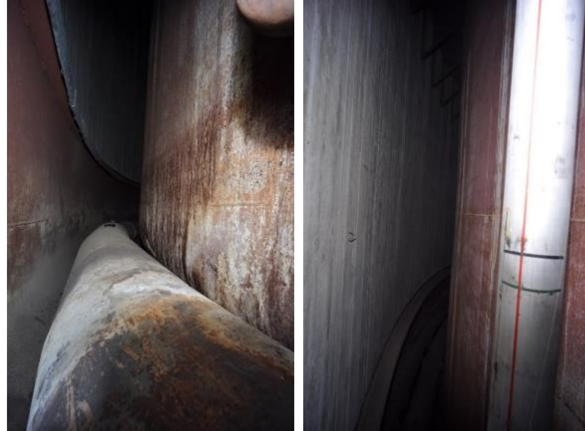
South Riser Facing West
