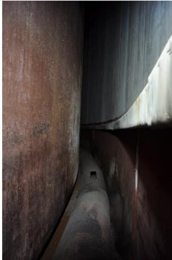
East Riser Facing North
