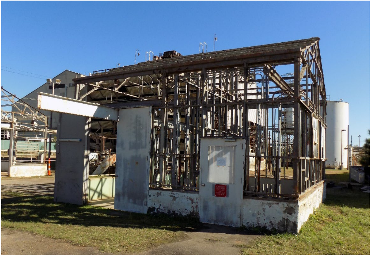
Figure 2. Building 480-3D (Looking South) After Asbestos Abatement
