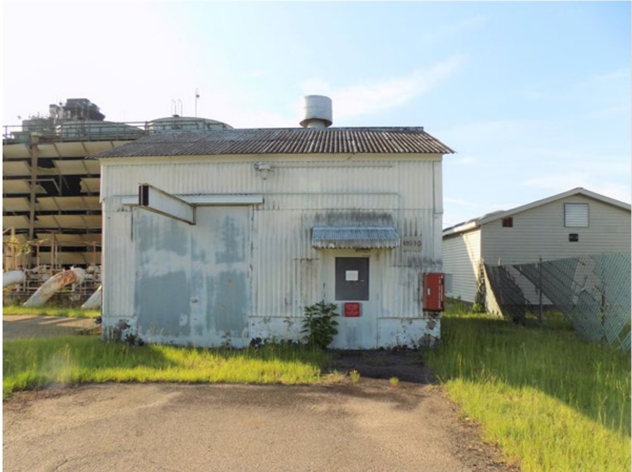
Figure 1. Building 480-3D (Looking South) Before Asbestos Abatement
