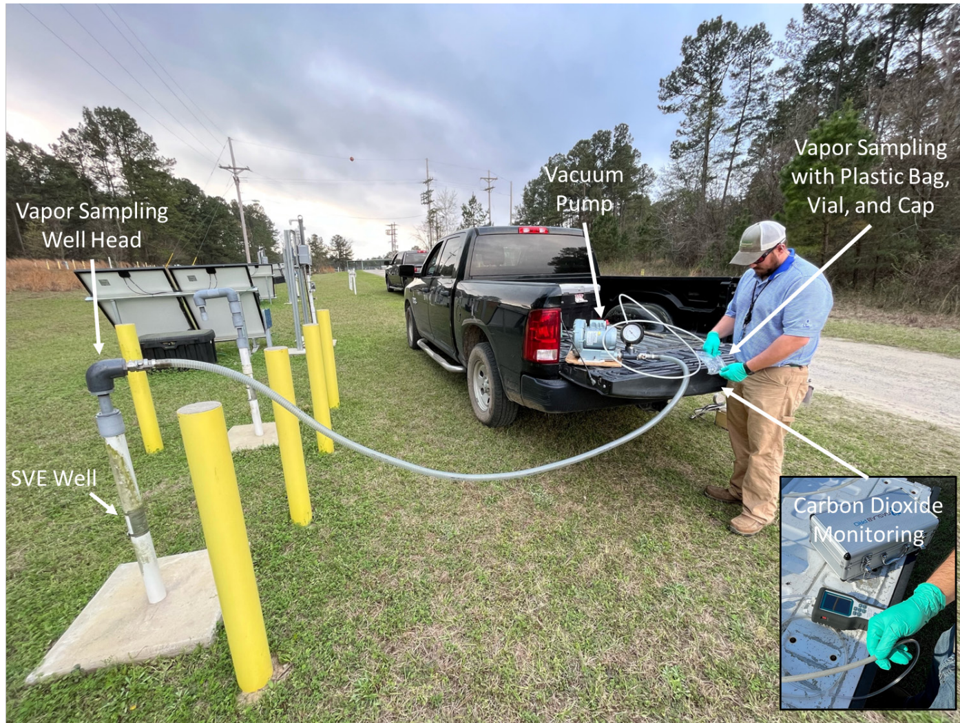
Figure 3. Diagram of Collecting a Soil Vapor Sample from an SVE Well using a Vacuum Pump.
