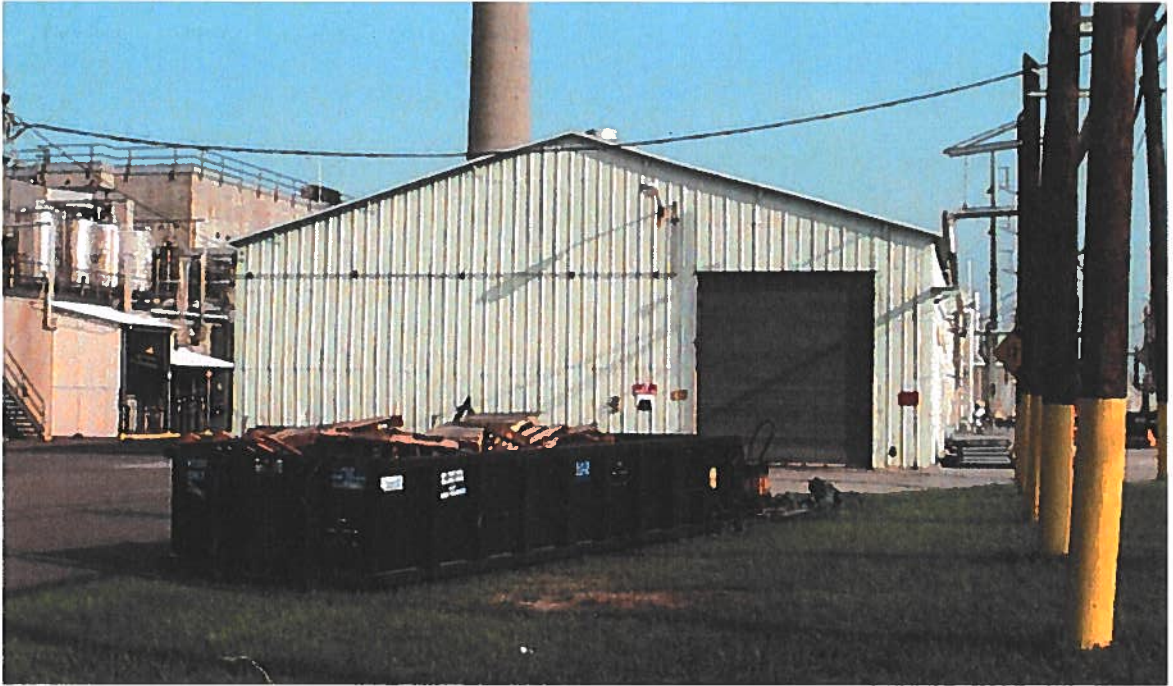
Photo 1 – Building 232-1H Before Decommissioning (Looking North)
