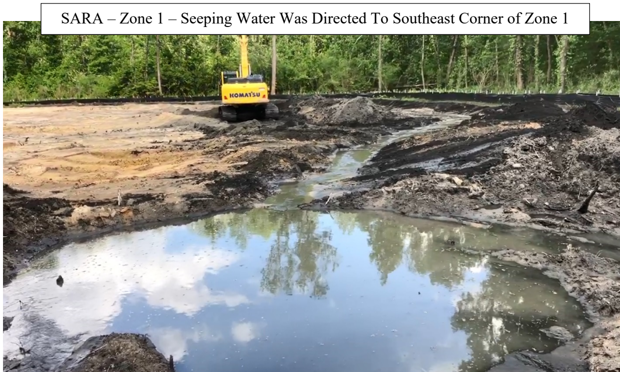
Figure 7. SARA Phase II Excavation of Ash in Zone 1
