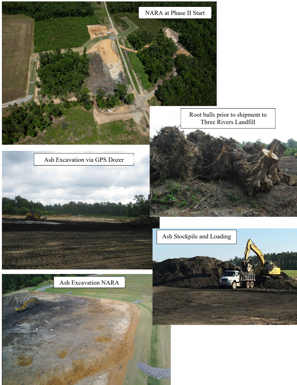
Figure 11. NARA Phase II- Clearing and Grubbing and Excavation Activities
