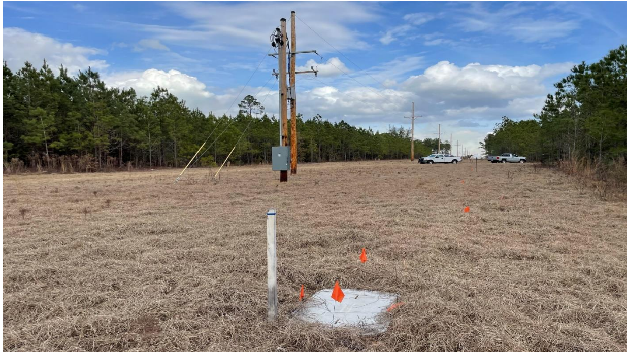
Photo 8: View of utility poles and buried utility markers adjacent south of the proposed access/utility easement, facing northeast.
