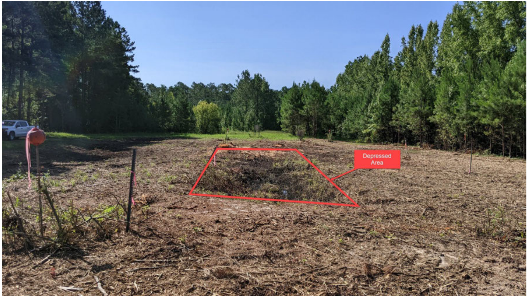
Figure 2-7. Depressed Area within LRP 131-1L Subunit
