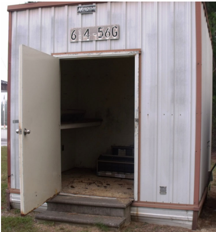
614-56G Equipment Shed New Ellenton Barricade
