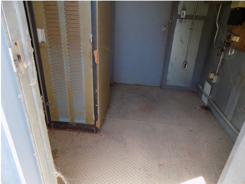
686-1G – Dam Service Building (L Lake)
