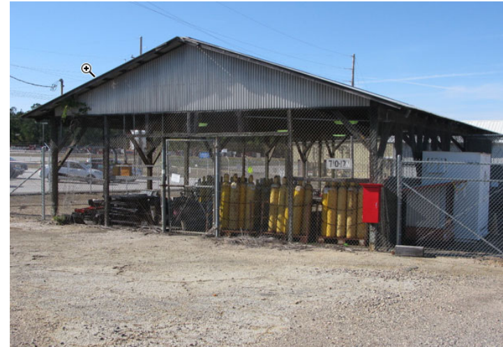
710-12N Tire Storage Canopy
