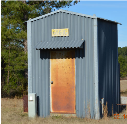
686-1G – Dam Service Building (L Lake)
