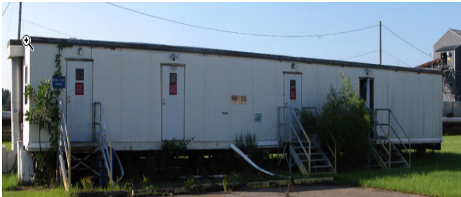
484-2D Coal Handler's Change House
