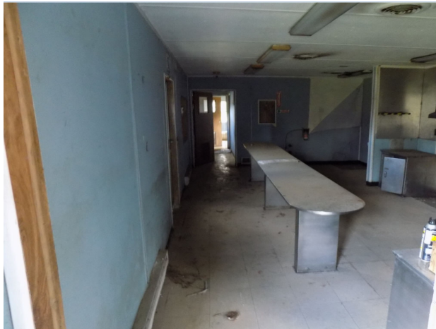
484-2D Coal handler's Change House
