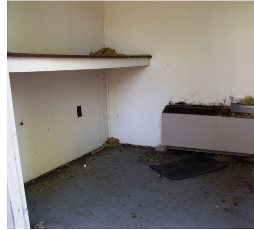
614-58G Equipment Shed East Talatha
