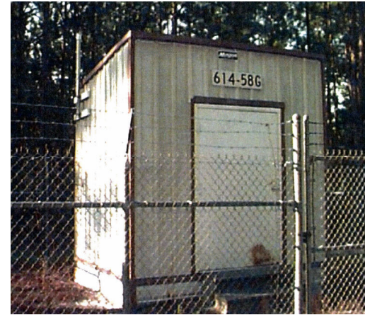
614-58G Equipment Shed East Talatha
