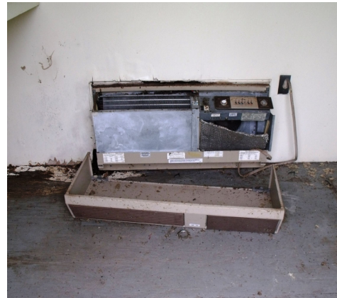
614-61G Equipment Shed Barnwell Barricade
