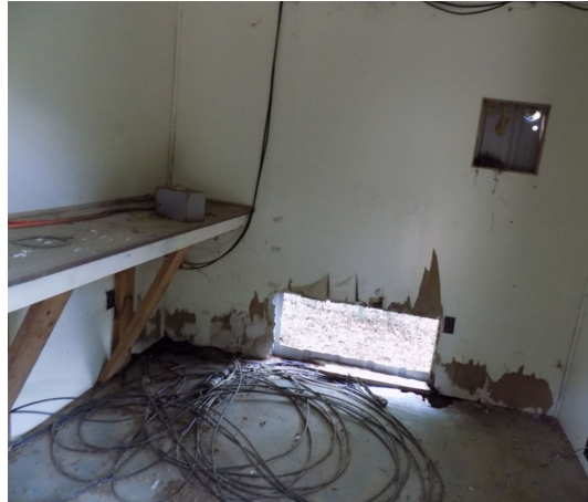
614-57G Equipment Shed Green Pond Road
