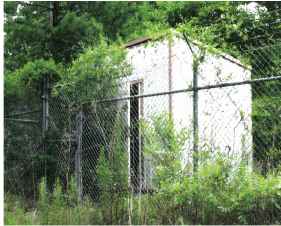
614-57G Equipment Shed Green Pond Road
