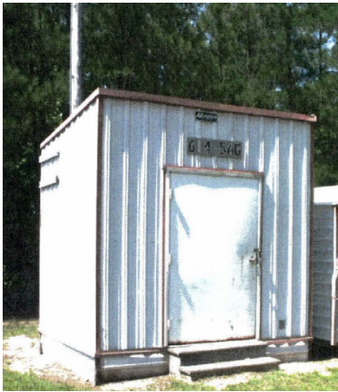
614-56G Equipment Shed New Ellenton Barricade
