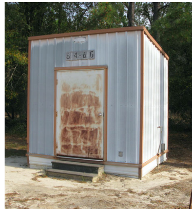
614-61G Equipment Shed Barnwell Barricade
