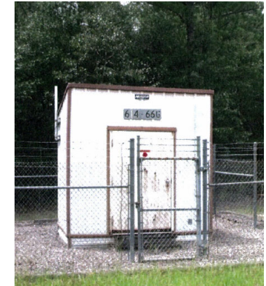
614-66G Equipment Shed Highway 21 / 167
