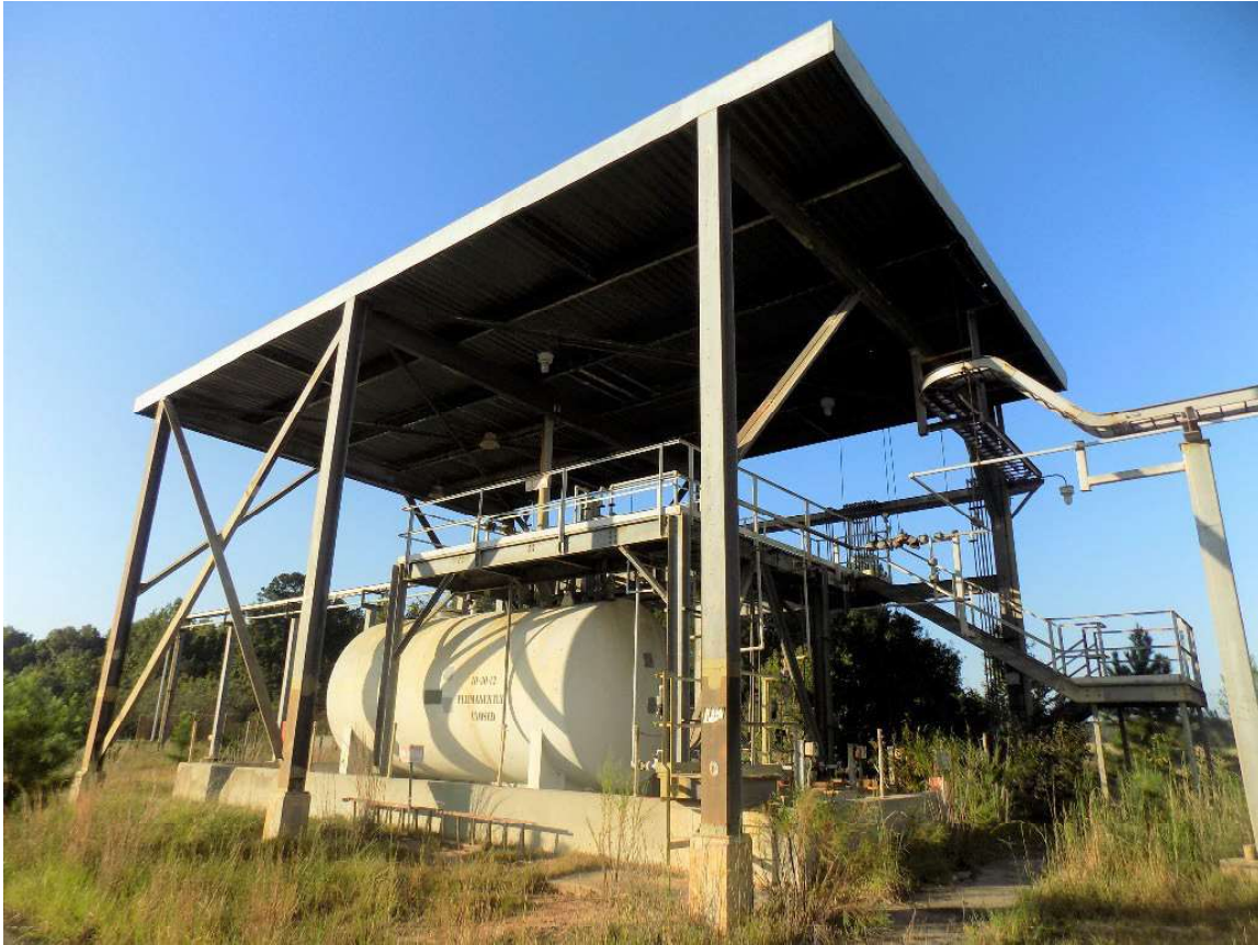
Figure A-1. Building 454-D (Looking East) Before
