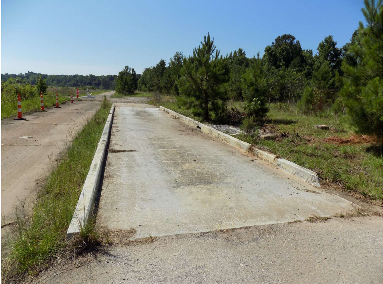
Figure A-5. Building 454-1D (Looking South) After
