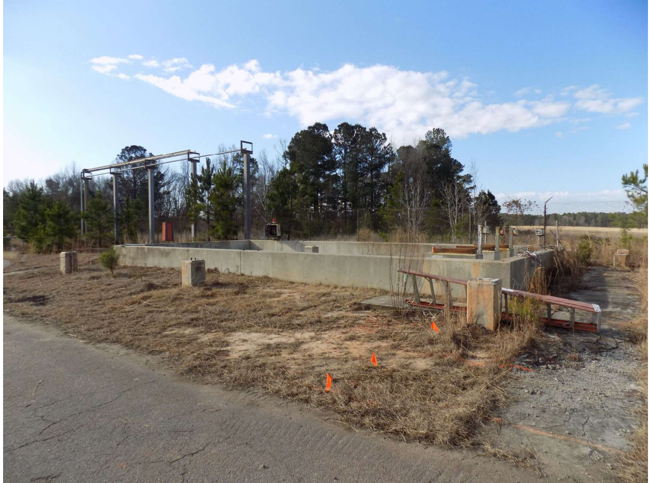
Figure A-2. Building 454-D (Looking East) After Partial Decommissioning by CRO
