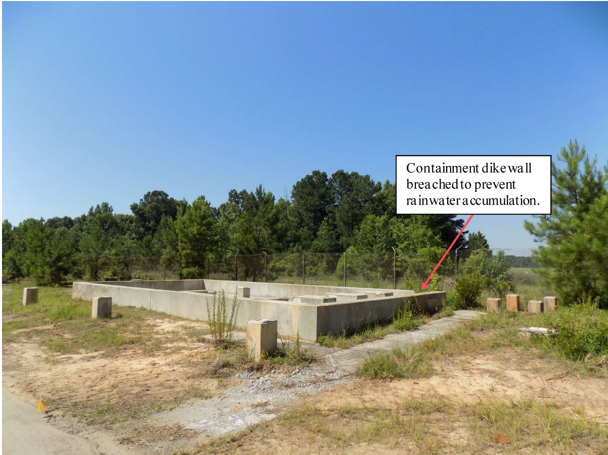
Figure A-3. Building 454-D (Looking East) After Final Decommissioning
