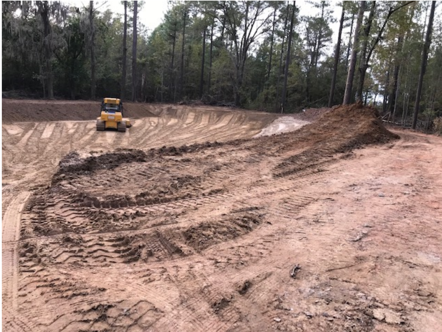
Figure 11. Placement of Common Fill in Support of GOSB OU Closure
