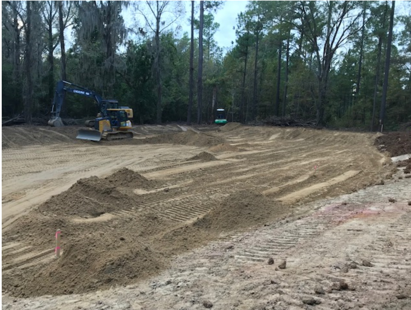
Figure 12. Spreading and Compacting Common Fill in Support of GOSB OU Closure
