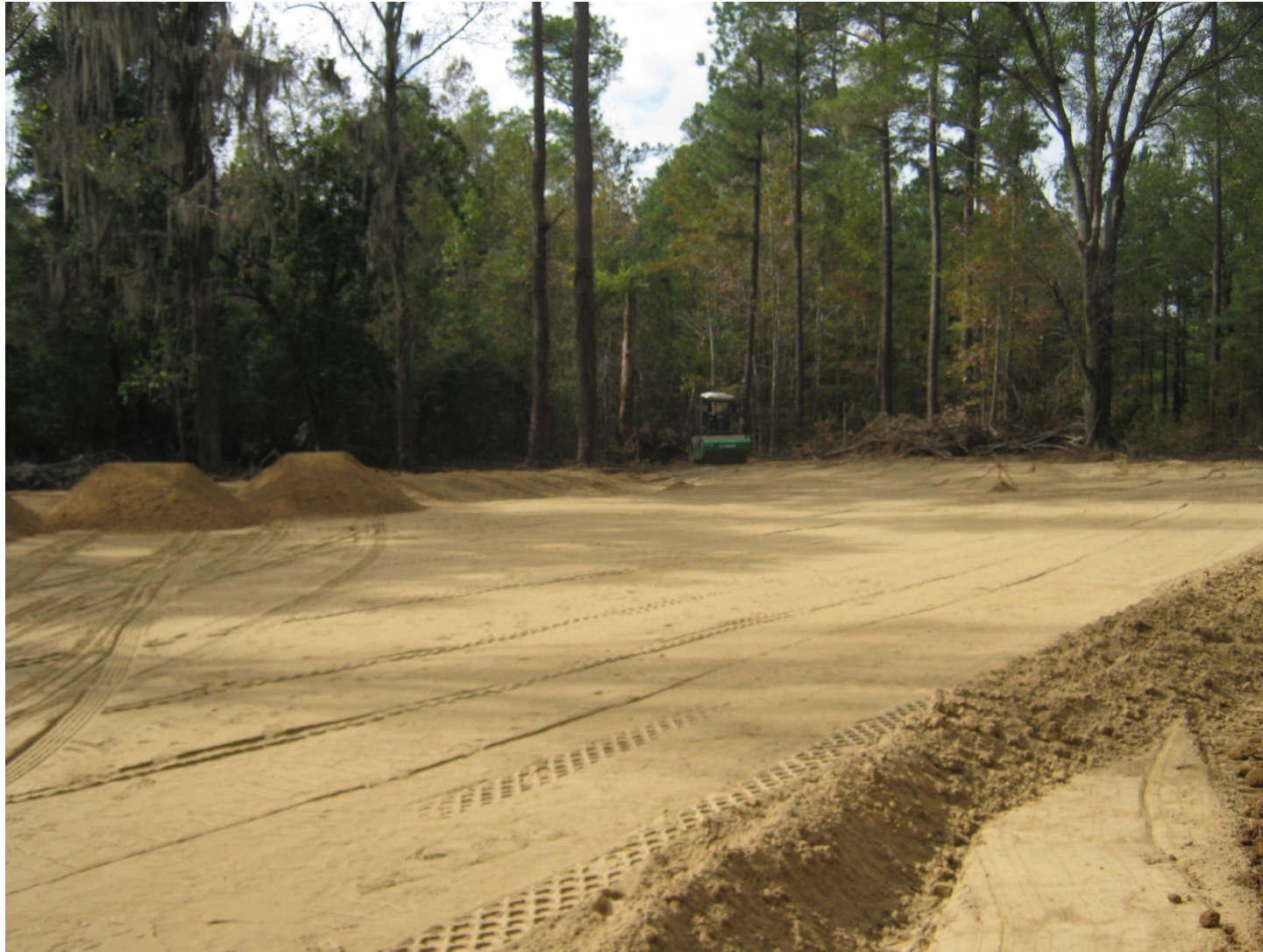
Figure 13. Compacted Common Fill at GOSB OU Prior to Mounding
