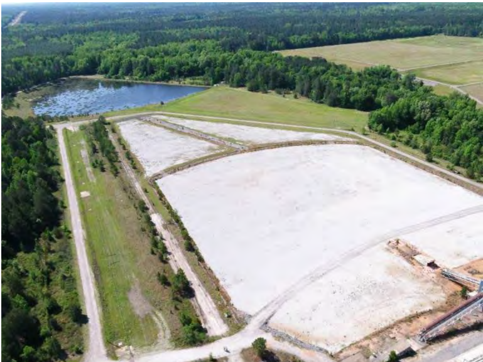
Figure 31. Photograph After Completion of the Soil Neutralization at the 484-17D DCSA
