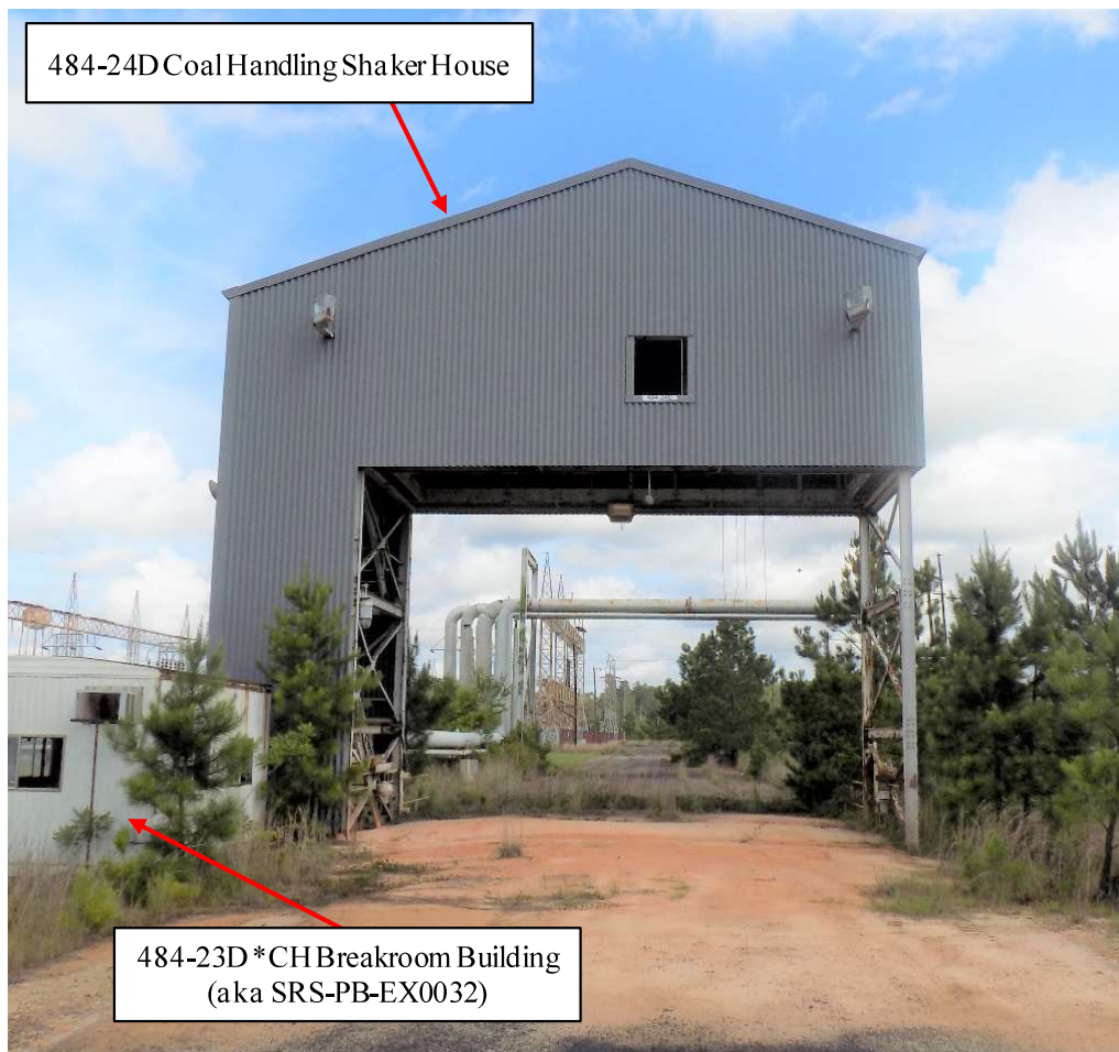
Figure 3. Building 484-24D, Coal Handling Shaker House (Looking North)
