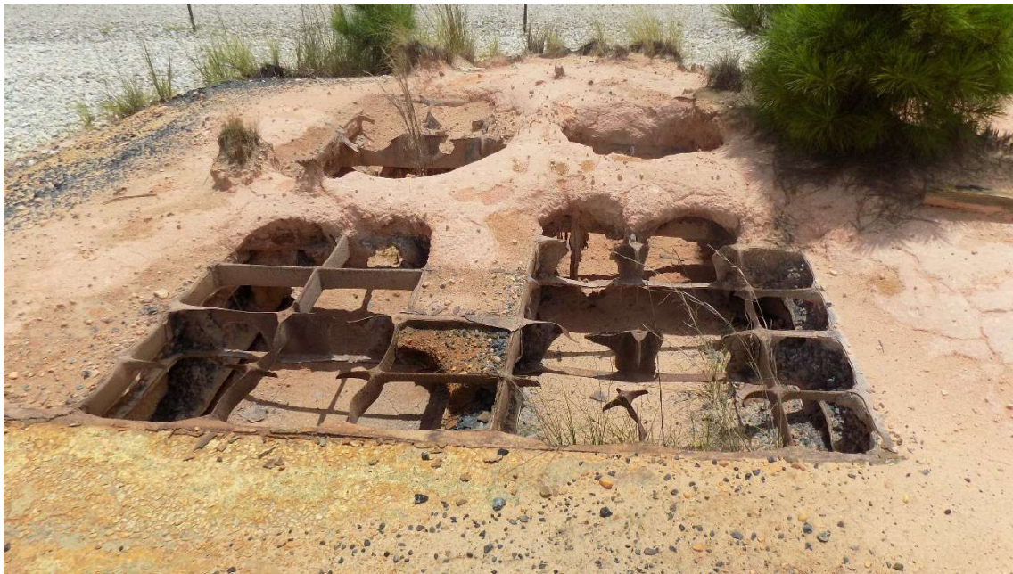
Figure 13. Reclaim Hopper South of 484-22D Crusher House
