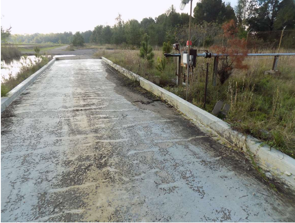
Figure 27. Building 454-1D, D-Area Diesel Fuel Unloading Facility (Looking South)
