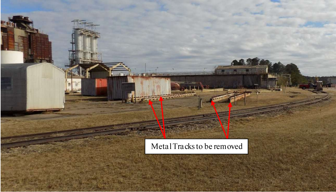
Figure 35. Ancillary Metal Tracks to be Removed
