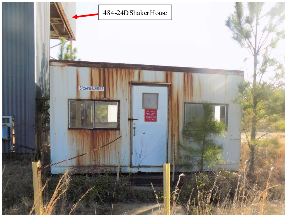
Figure 5. 484-23D Coal Handling Breakroom Building (aka SRS-PB-EX0032)
