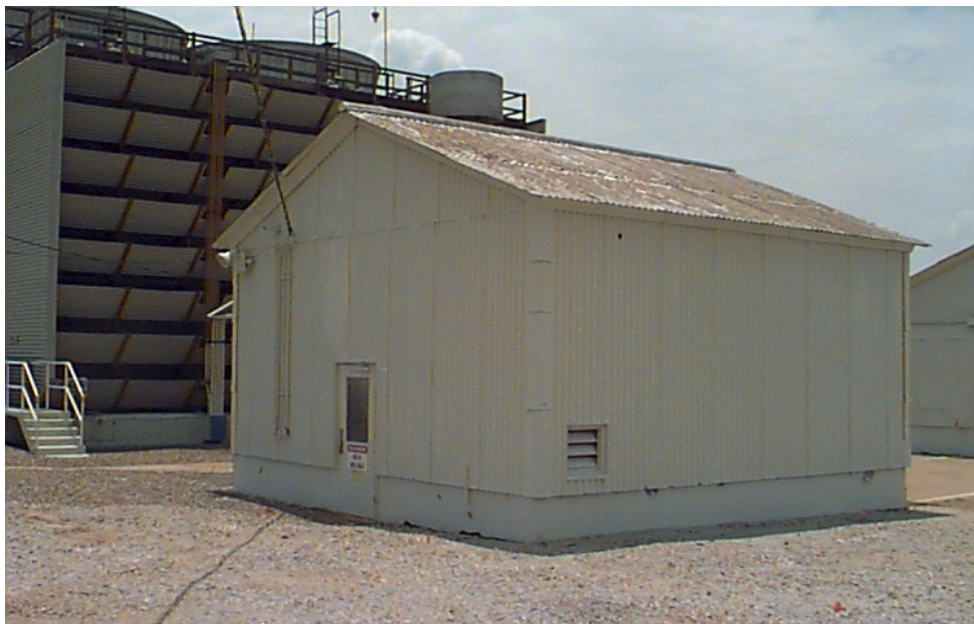
Figure 6. Building 482-2D, Cooling Tower Switchgear Building
