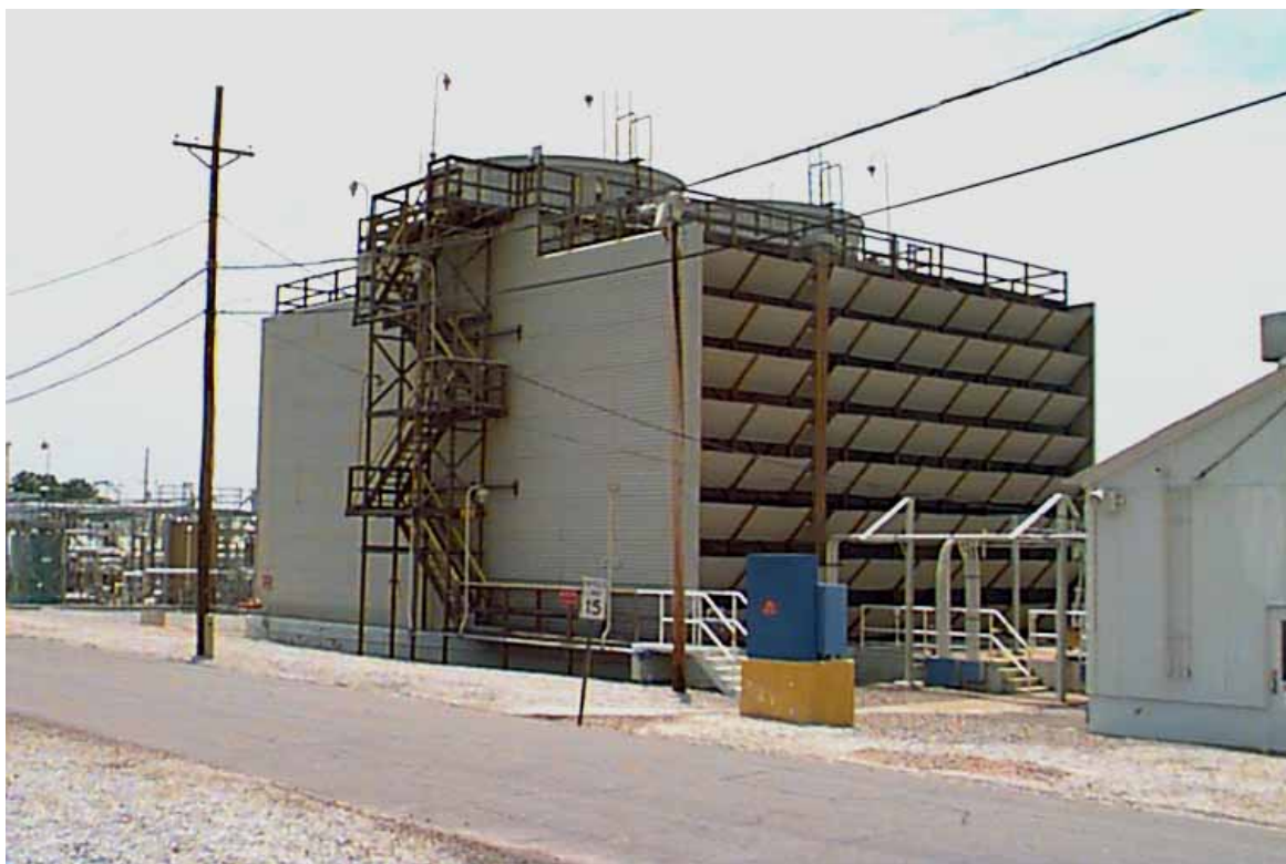
Figure 1. Building 485-D, D-Area Cooling Tower (Looking Southwest)
