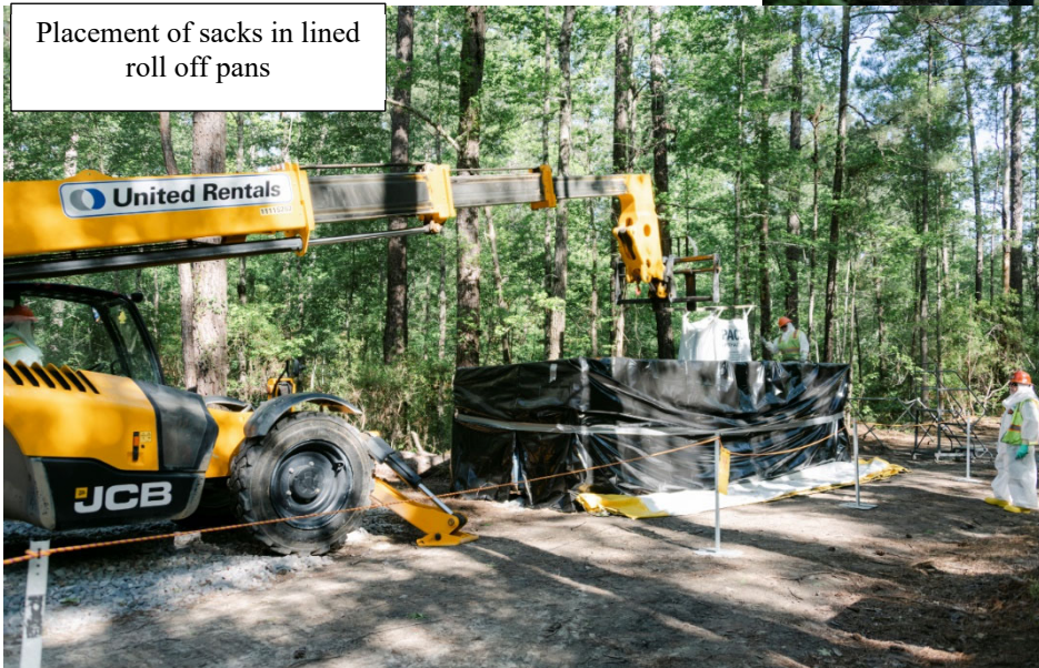
Figure 15. Excavation of R-Area Discharge Canal Sediments
