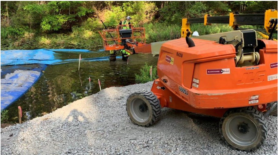
Figure 10. Photos of Equipment - Telehandler
