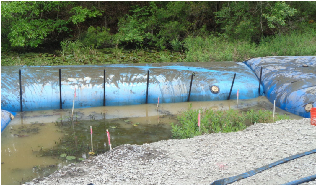
Aqua Barriers Inflated with Canal Water
