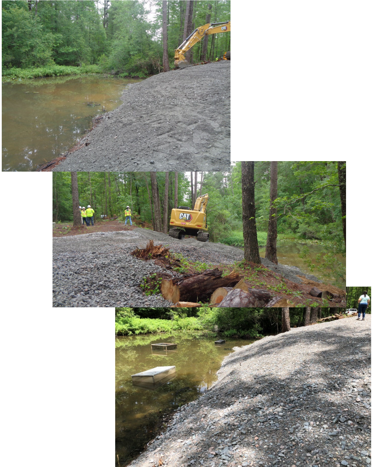
Figure 18. Final Grading and Final Acceptance Inspection
