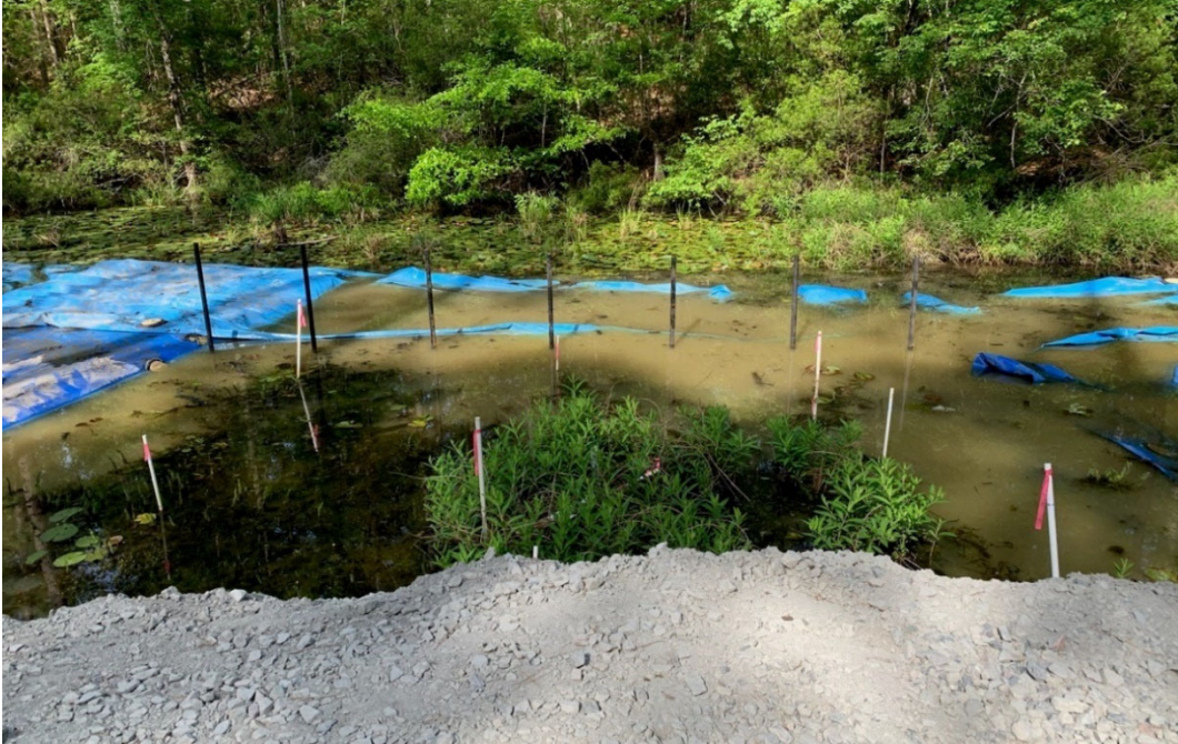
Aqua Barriers Inflated with Canal Water
