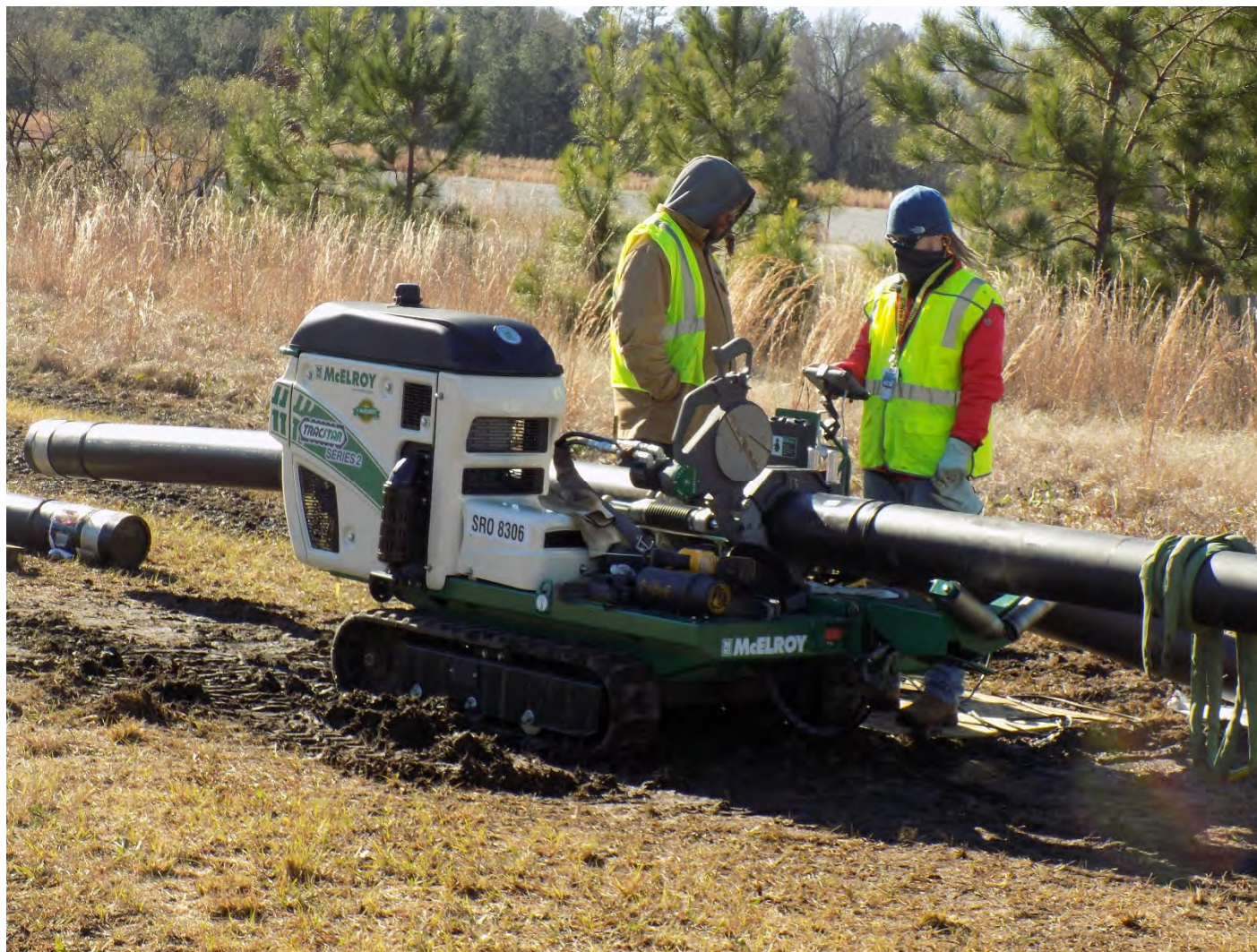
Figure 10. D-Area Treatability Study Pipeline Installation
