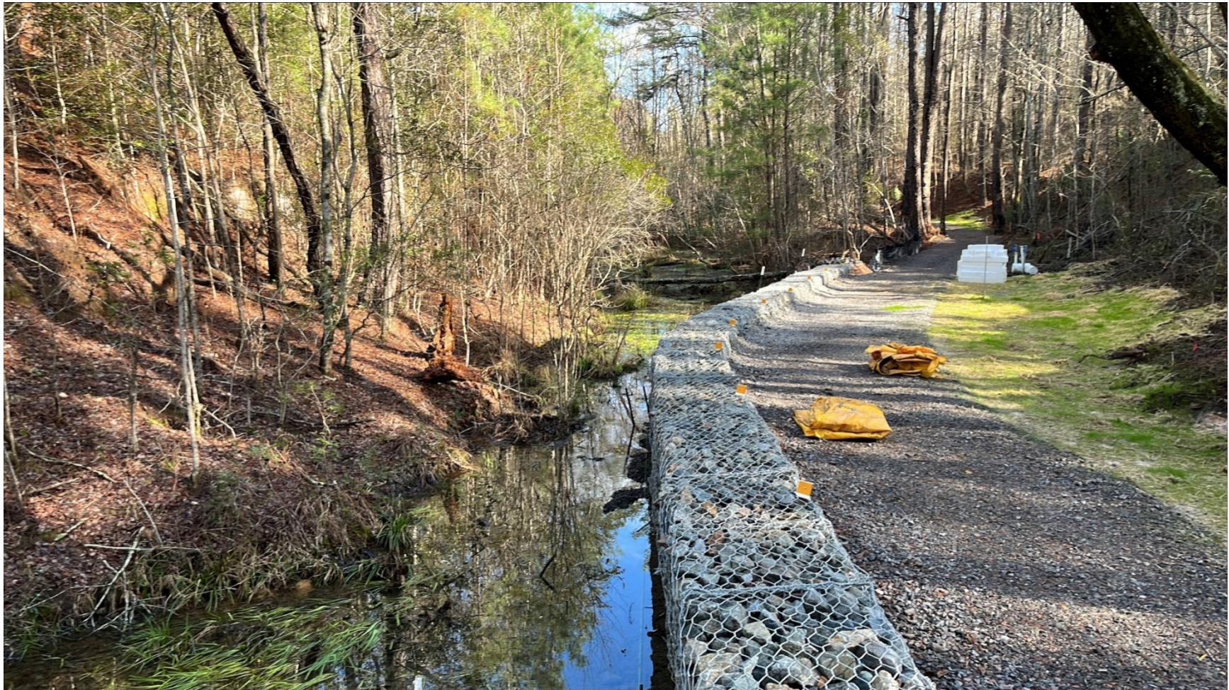
Figure 30. Steel Creek Sampling Access Road Completed in January 2023
