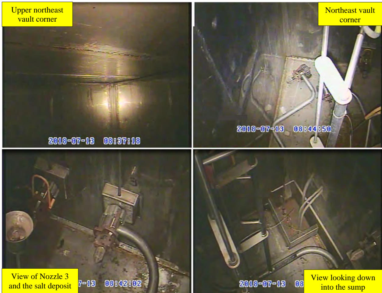
Figure 9.0-2: Views of the FDB-6 Vault Interior
