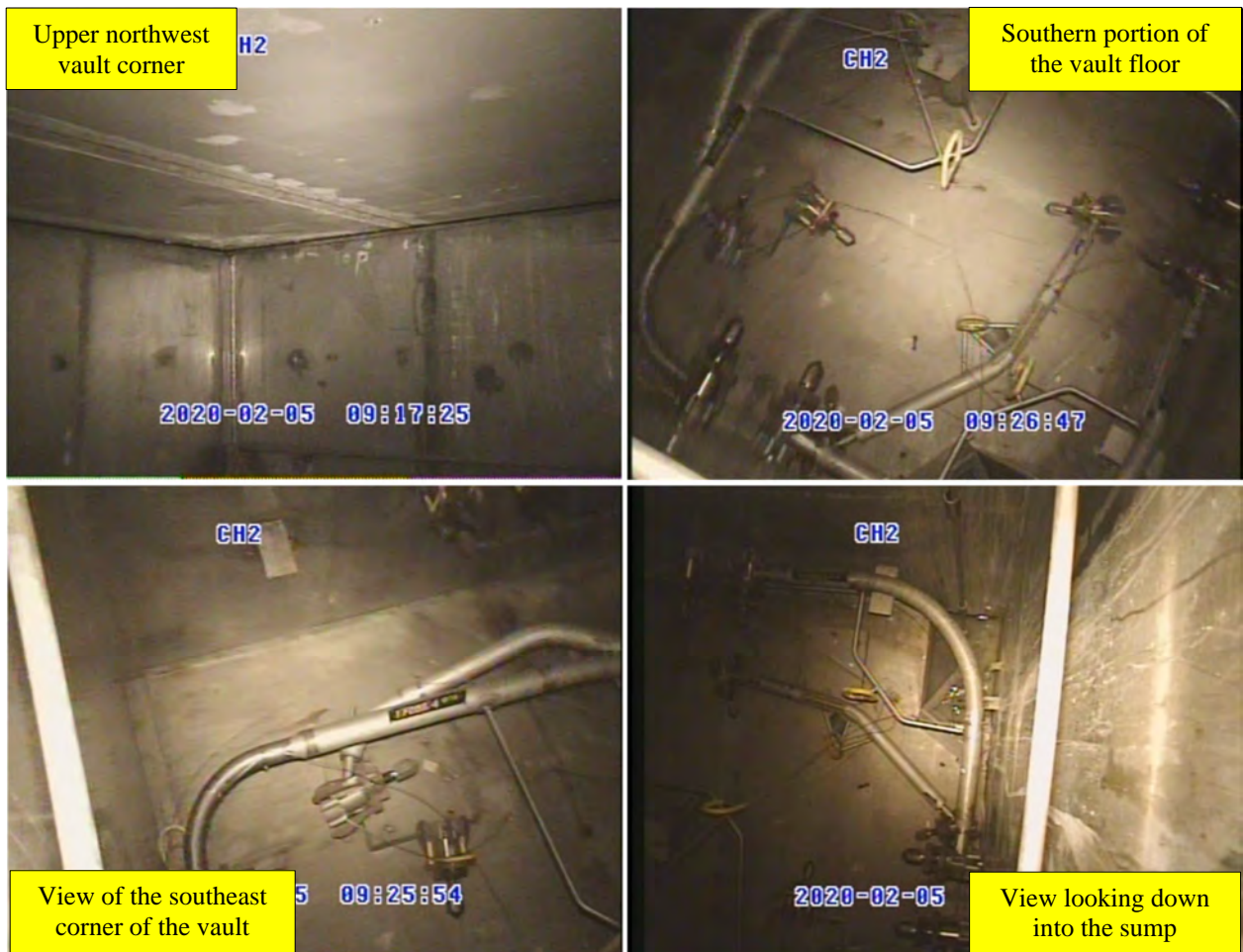
Figure 9.0-1: Views of the FDB-5 Vault Interior
