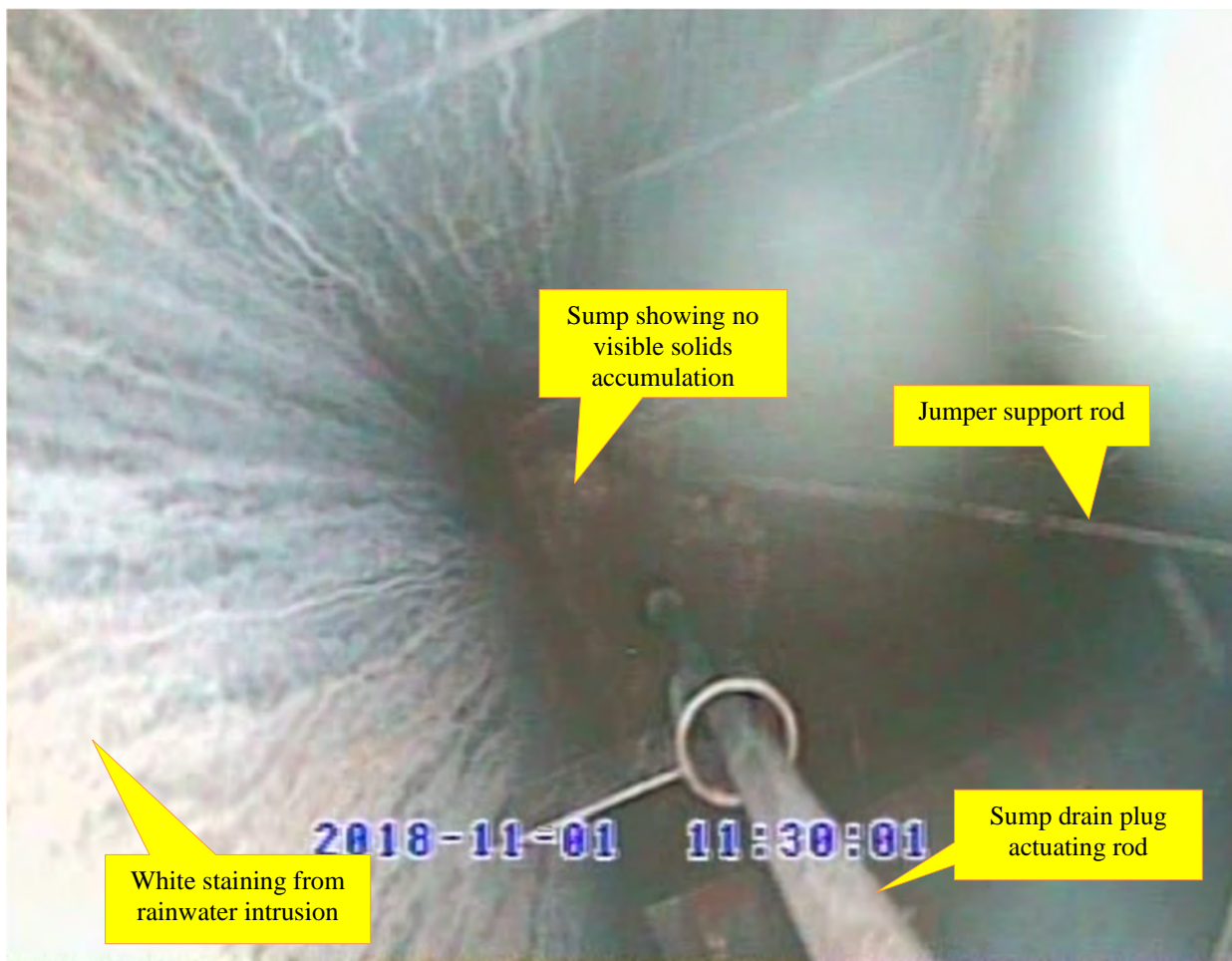
Figure 2.4-1: View Looking Down at the FDB-5 Sump (November 2018)
