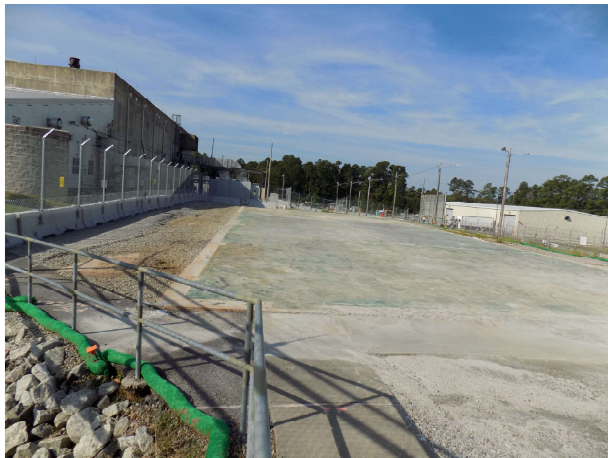
Figure 2: 233-22H Looking West-Northwest (After)
