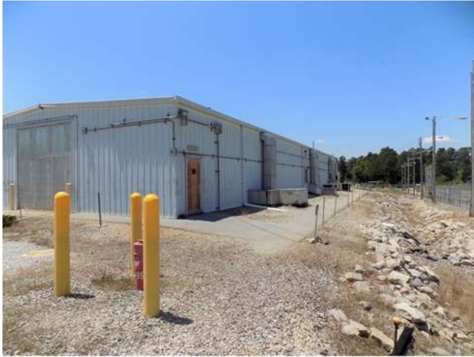
Figure 3: 233-22H Looking West-Southwest (Before)
