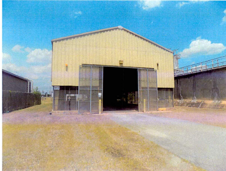
Figure A-1. Building 683-D (Looking East) Before
