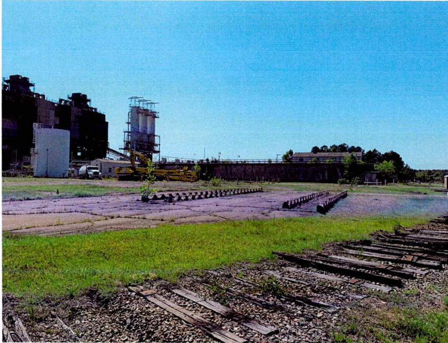
Figure A-7. Ancillary Metal Tracks (Looking Southeast) After
