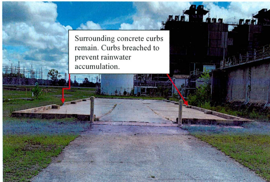
Figure A-3. Building 683-D (Looking East) After Final Decommissioning
