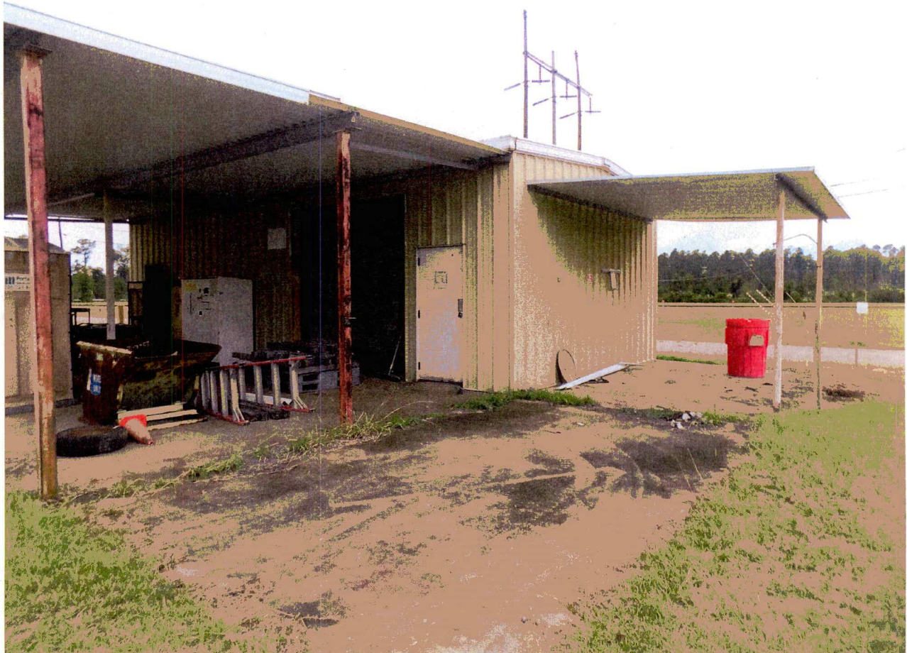
Figure 1: Building 484-7D (Looking North) Before
