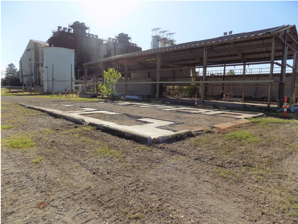
Figure A-2. Building 710-16D (Looking Southeast) After Decommissioning
