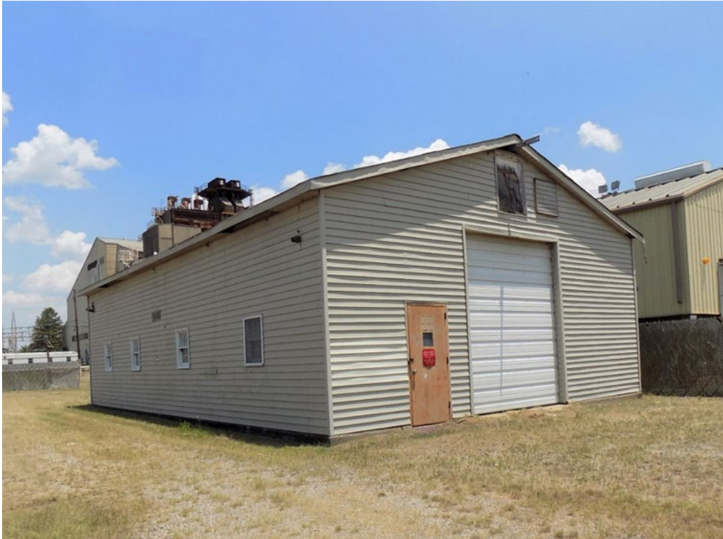
Figure A-1. Building 710-16D (Looking Southeast) Before Decommissioning
