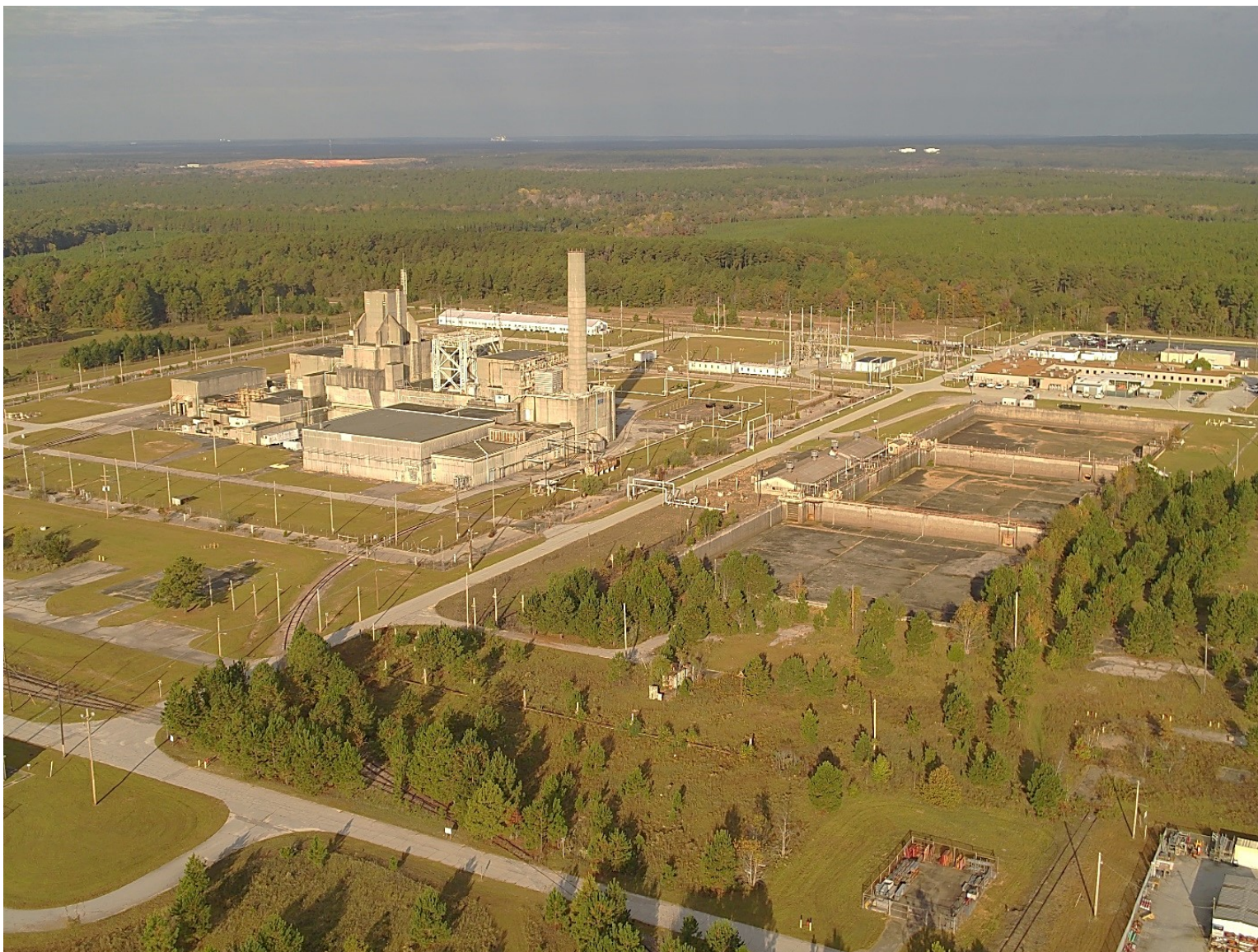
Figure C-5. Current Aerial Photograph of CAOU (2023)
