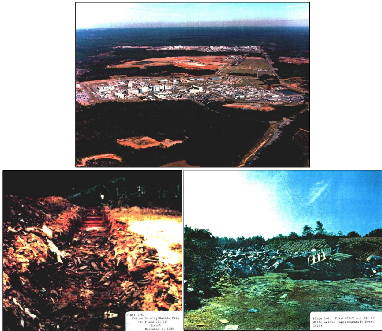
Figure F-3. Photos of F-Area Burning/Rubble Pits during Operational Period
