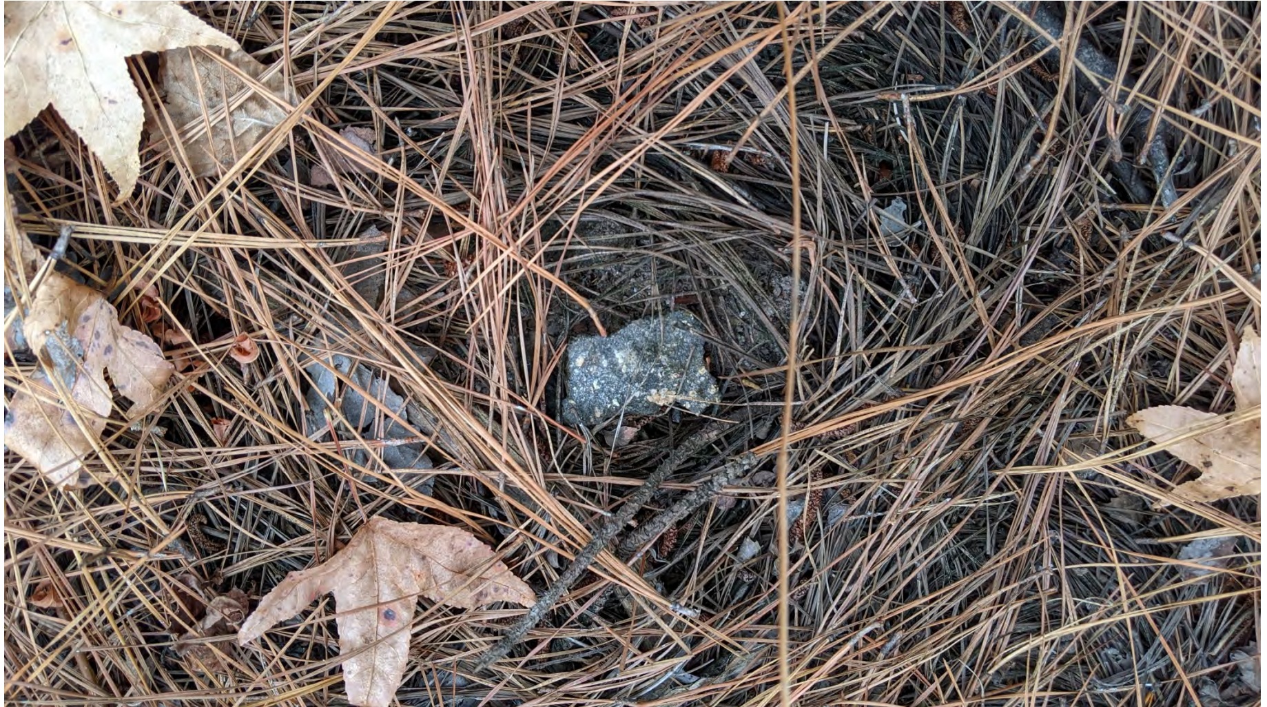
Figure 9. Asphalt Debris Observed at LRP 131-1L During December 2021 Walkdown
