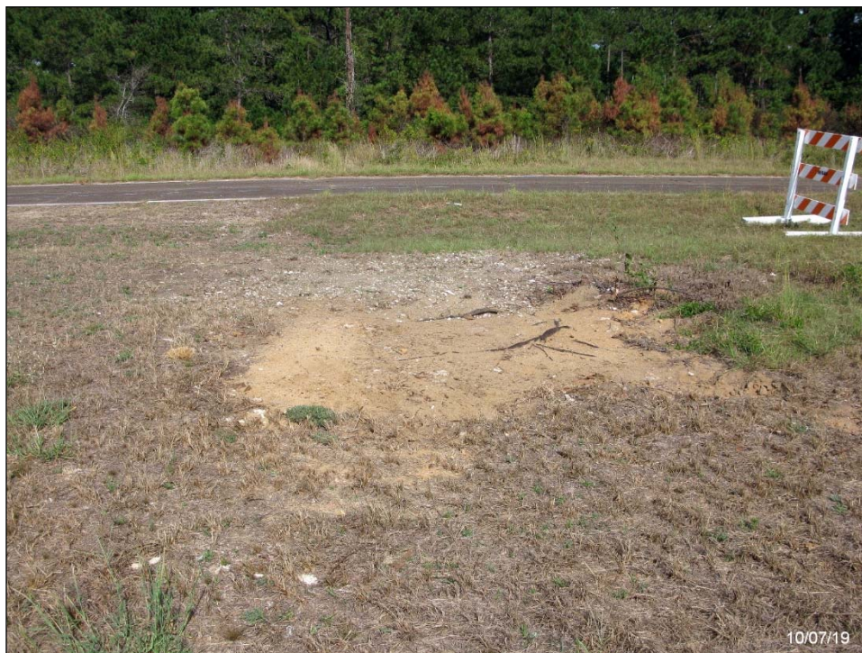
Figure 8 – 614-65G After Demolition
