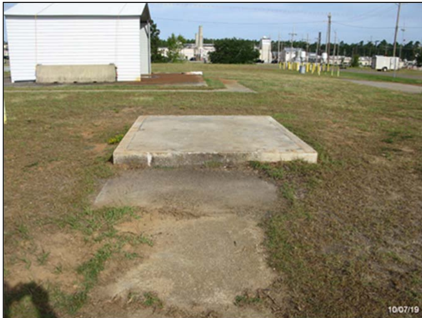
Figure 2 – 614-1A After Demolition
