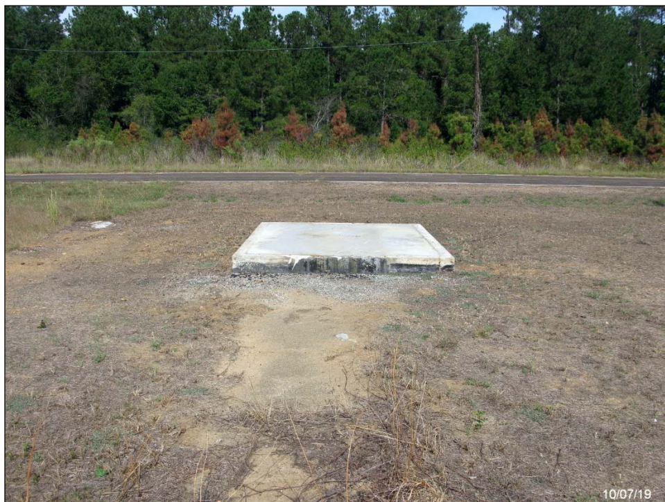
Figure 4 – 614-1D After Demolition
