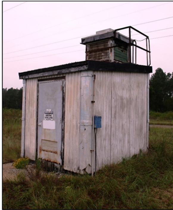
Figure 3 – 614-1D Before Demolition
