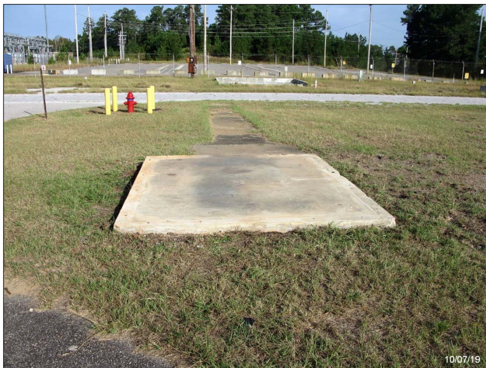
Figure 6 – 614-F After Demolition
