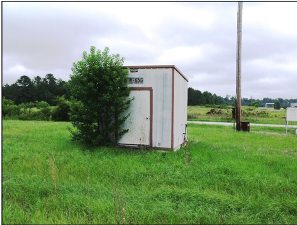
Figure 7 – 614-65G Before Demolition
