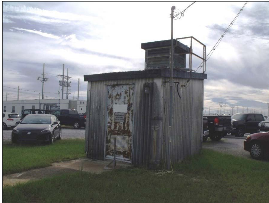
Figure 5 – 614-F Before Demolition
