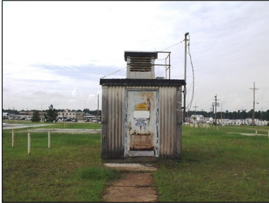
Figure 1 – 614-1A Before Demolition
