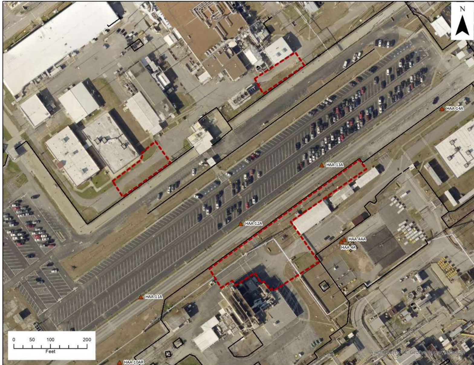
Figure 7: Aerial Photo of Parking Lot and Surrounding Area, H Area
