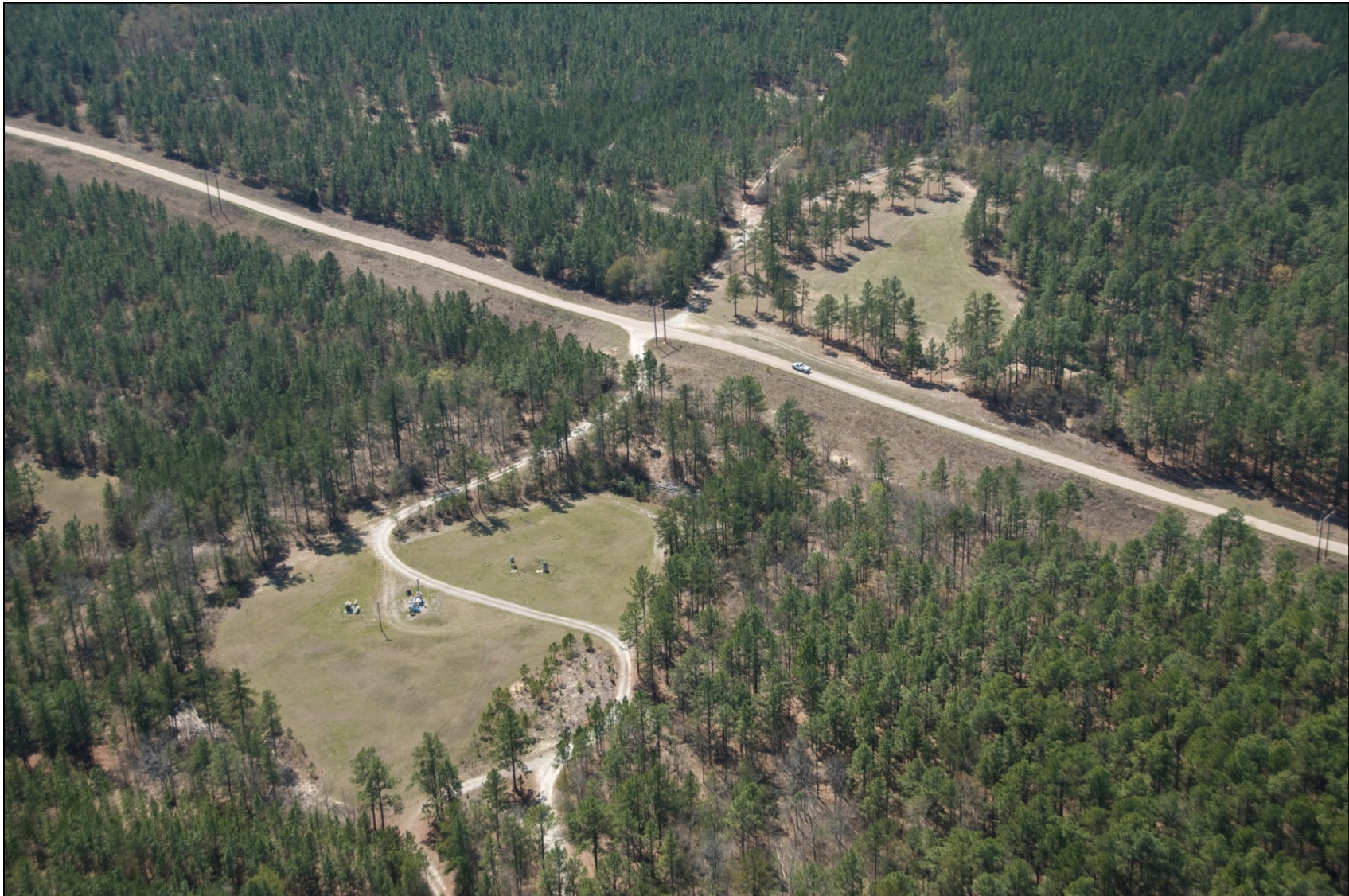
Figure C-9. Miscellaneous Chemical Basin after Final Action (2008)
