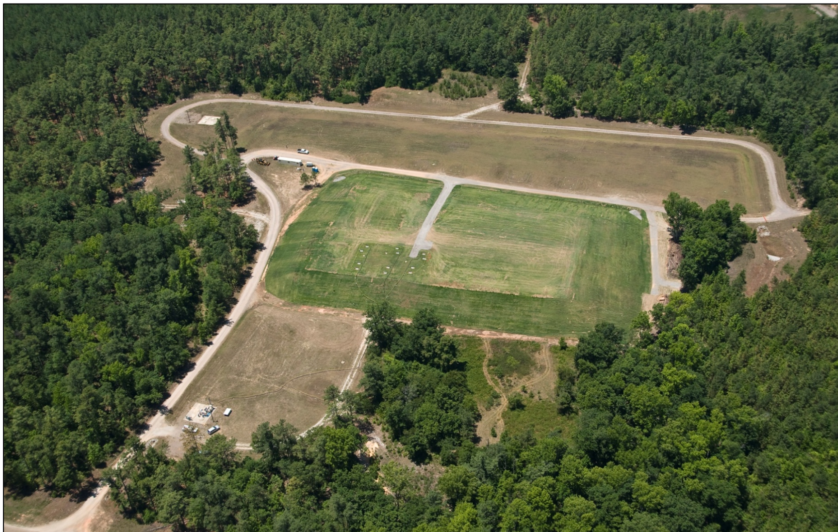
Figure C-6. A-Area Ash Pile and Underlying Trench Subunit after Final Action, with Installation of Trench Subunit SVE System (2008)
