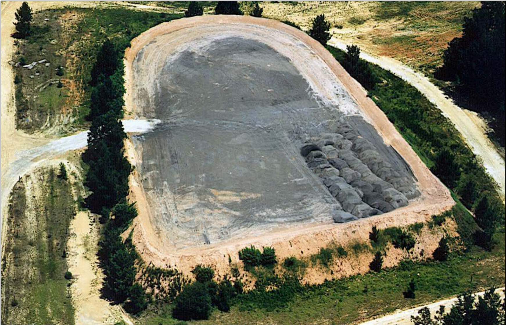
Figure C-4. A-Area Ash Pile and Underlying Trench Subunit during Operations (1981-1994)
