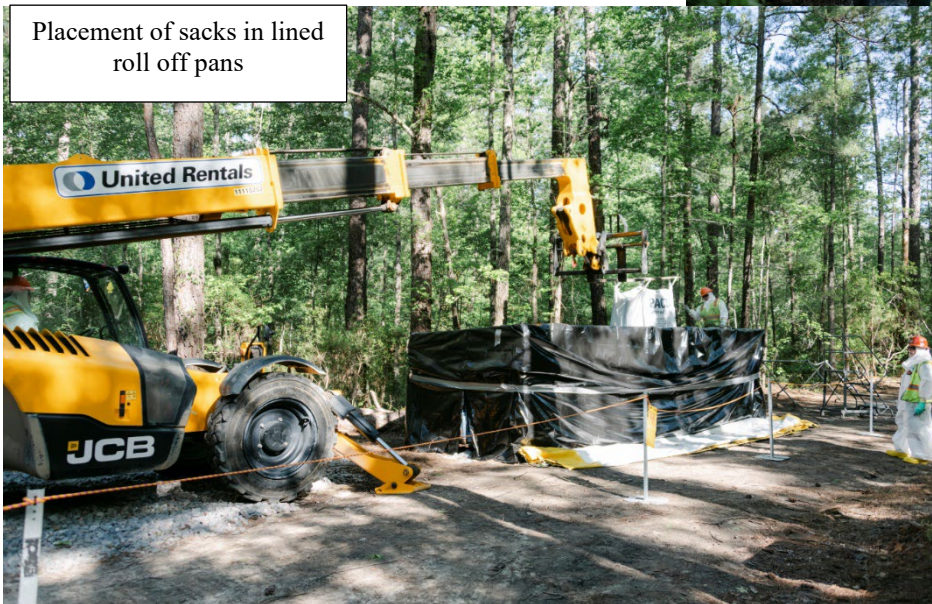
Figure 15. Excavation of R-Area Discharge Canal Sediments
