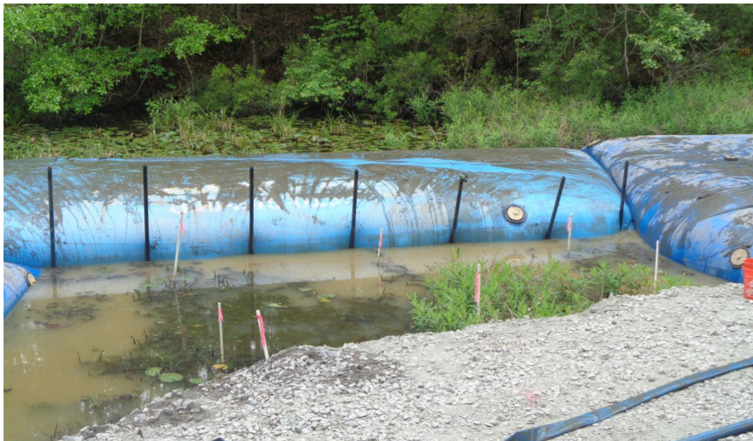
Aqua Barriers Inflated with Canal Water
