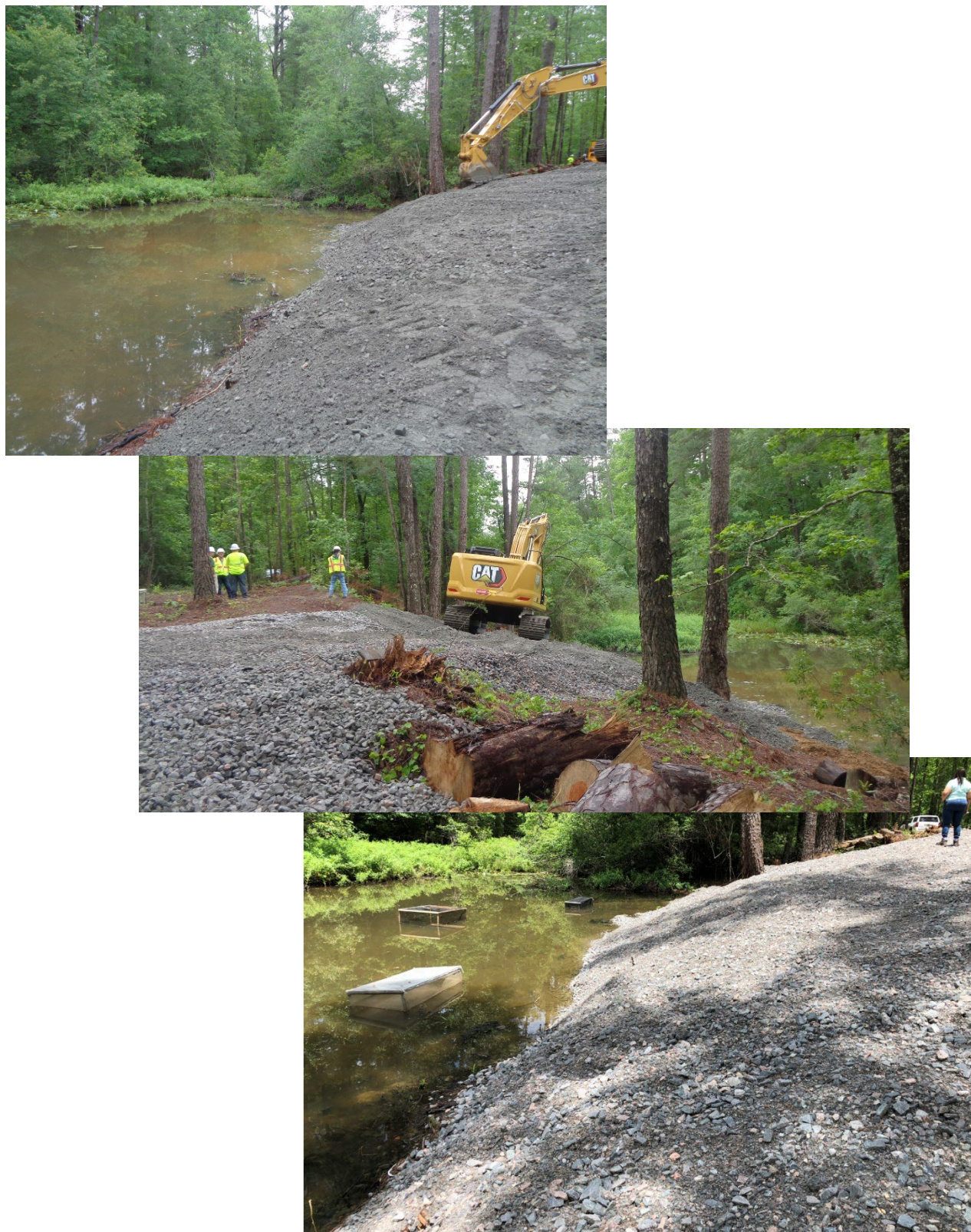
Figure 18. Final Grading and Final Acceptance Inspection
