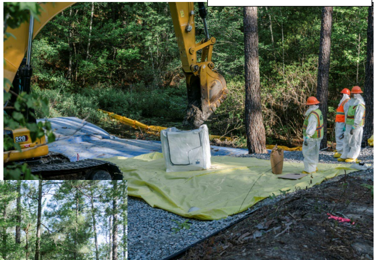
Placement of sediments in 1 cy double line sacks
