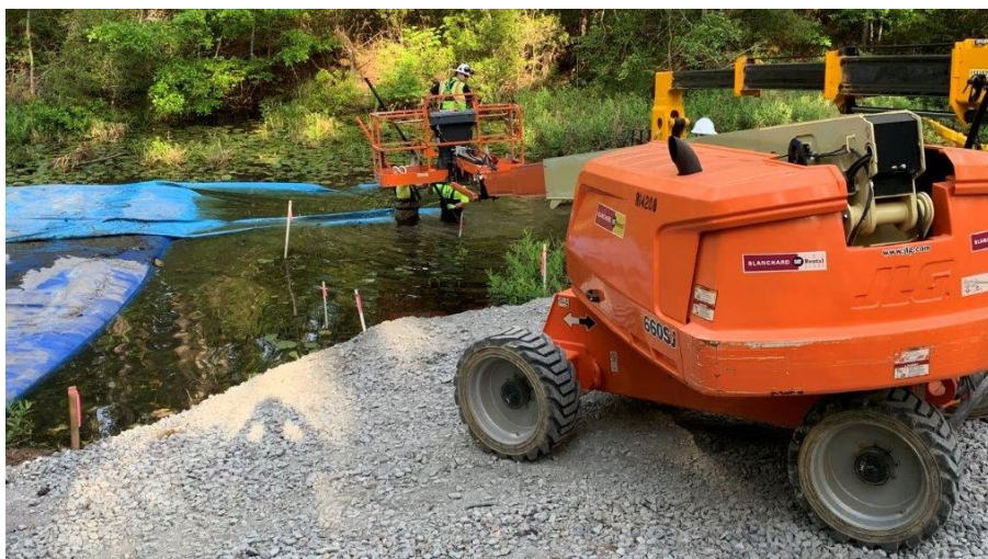
Figure 10. Photos of Equipment - Telehandler
