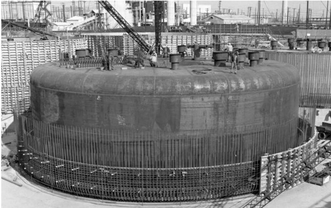
Type II Tank – Early Stage of Vault Construction
