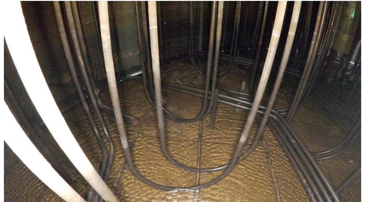
Northeast Quadrant from North
