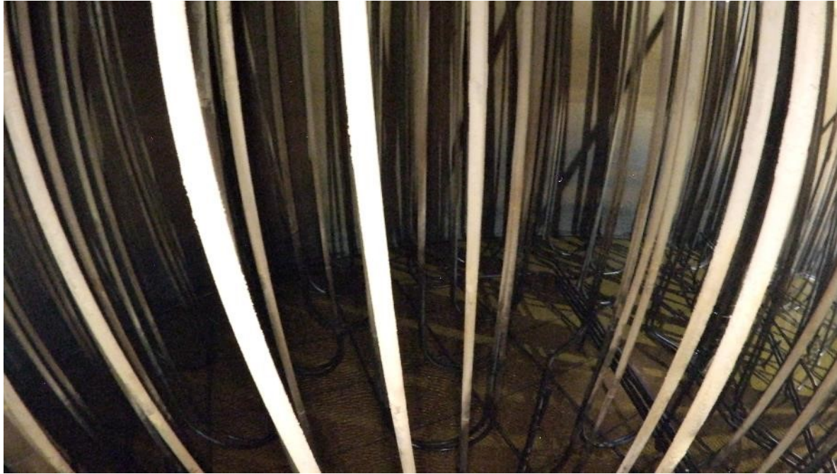
East Tank Wall
