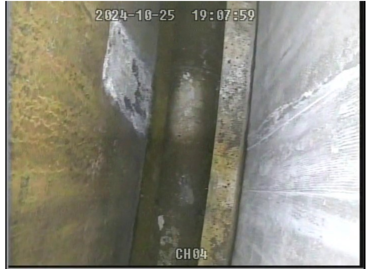
Northwest Quadrant (IP107)
