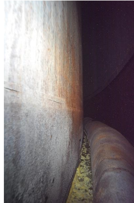
West Riser Facing South
