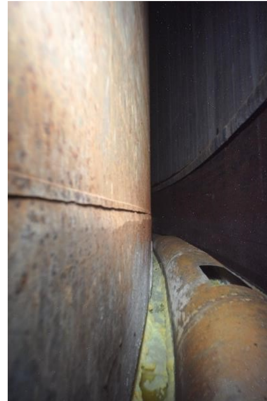
South Riser Facing East
