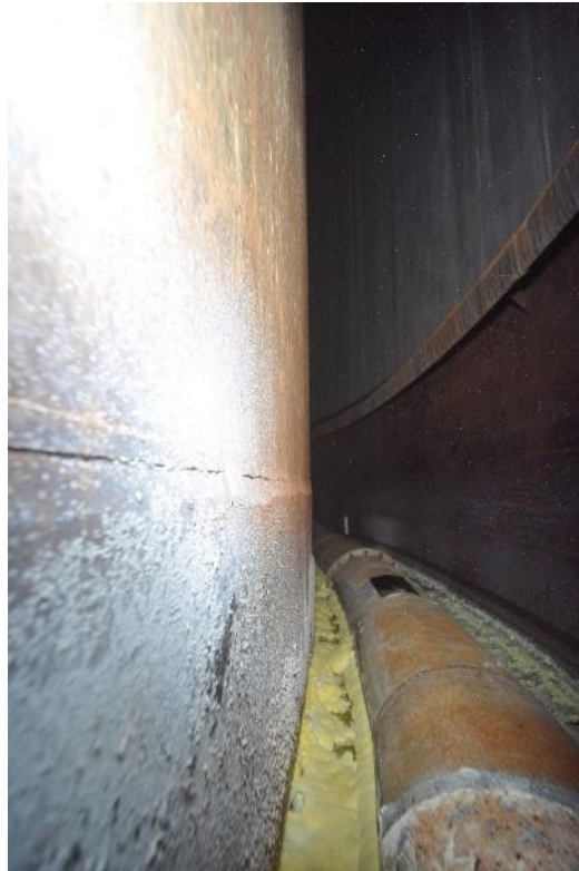
North Riser Facing West
