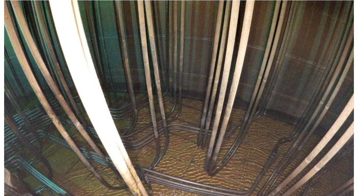
North Tank Wall
