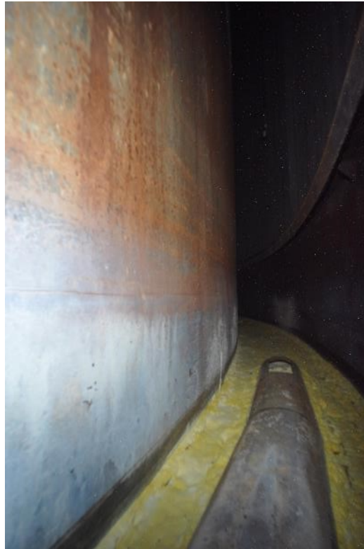
East Riser Facing North
