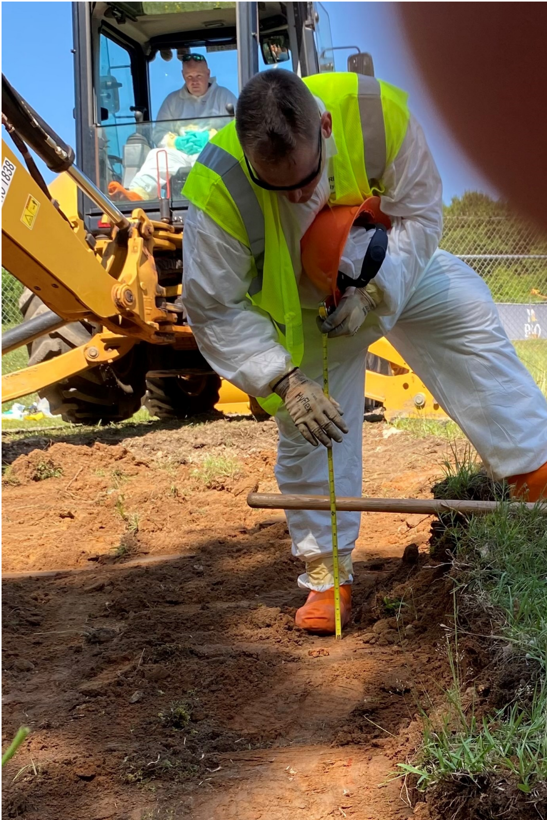
Figure 8. Verification of Excavated Depth at the 904-44G Spill Release Area (2024)
