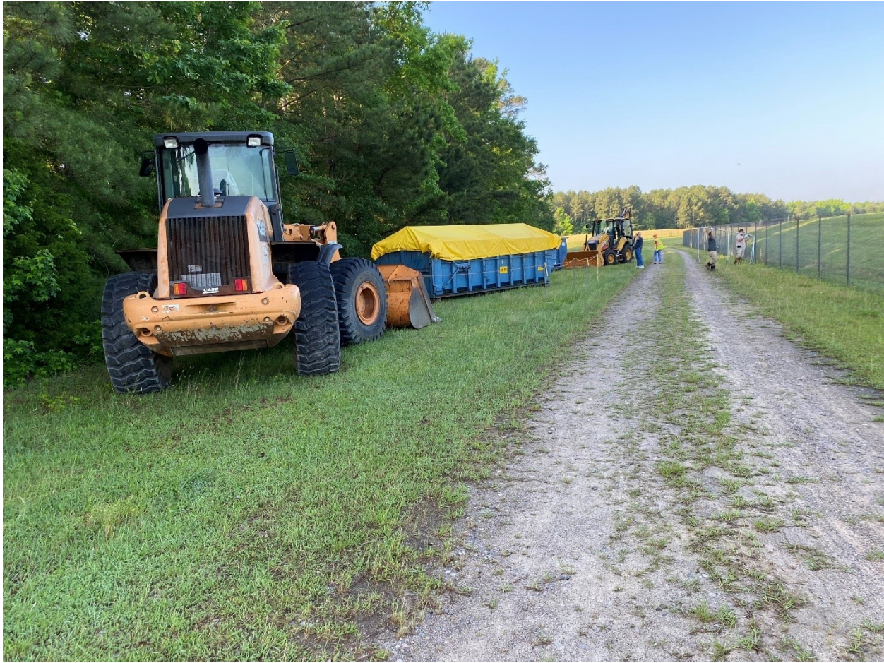
Figure 7. Containerization of Excavated Material from the 904-44G Spill Release Area (2024)
