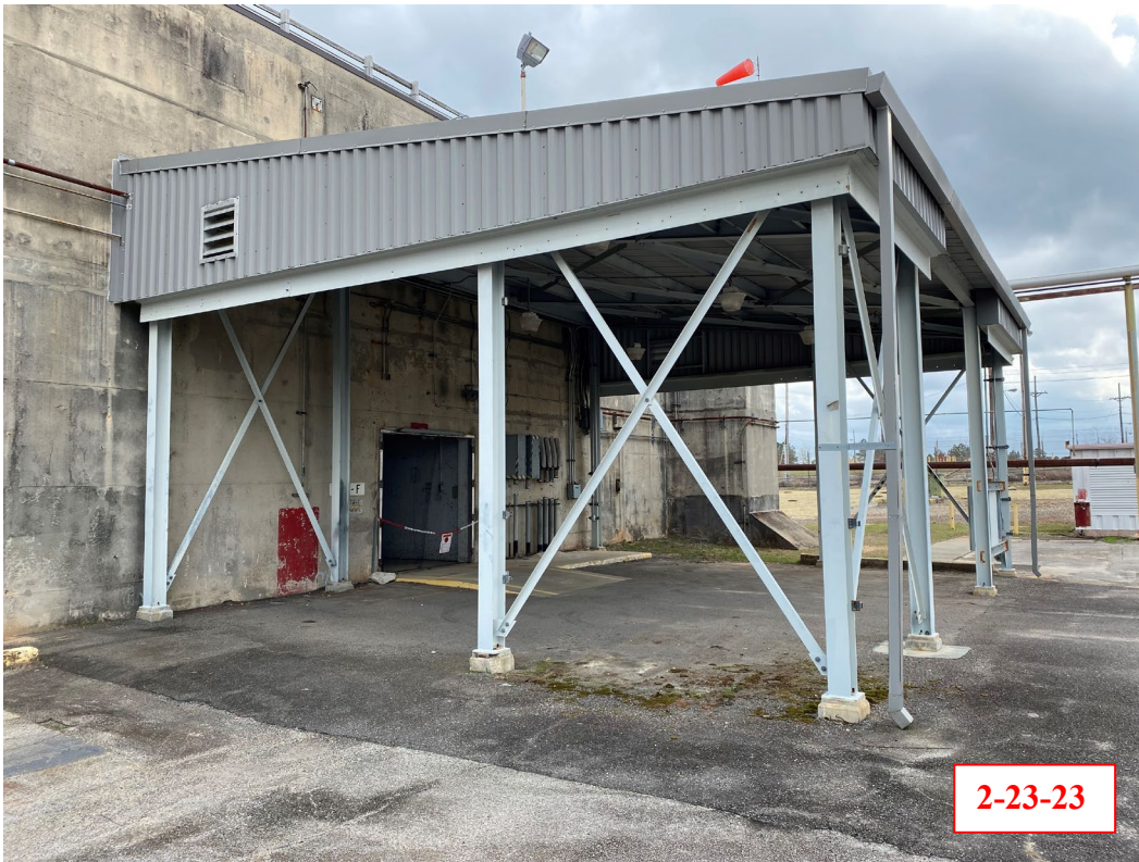
Figure B25 – West Covered Area of Building 235-F (Cleared, No Overhead Lines)
