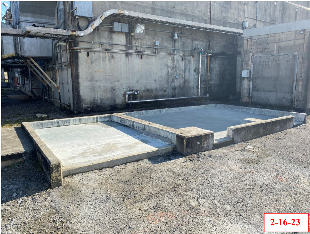
Figure B26 – Concrete Containment (281-28F) Northeast of Building 235-F
