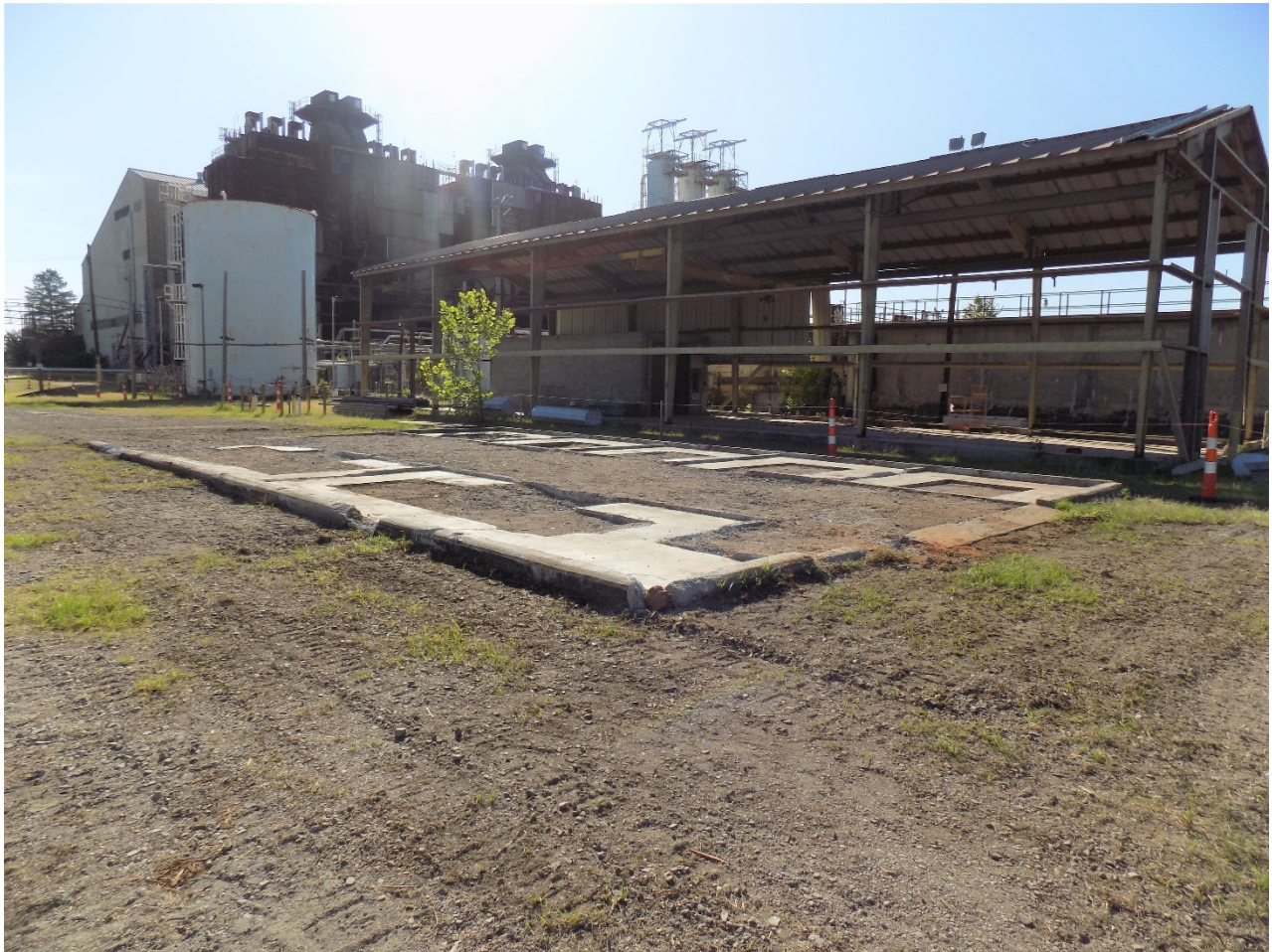
Figure 3. Building 710-16D (Looking Southeast) After Decommissioning
