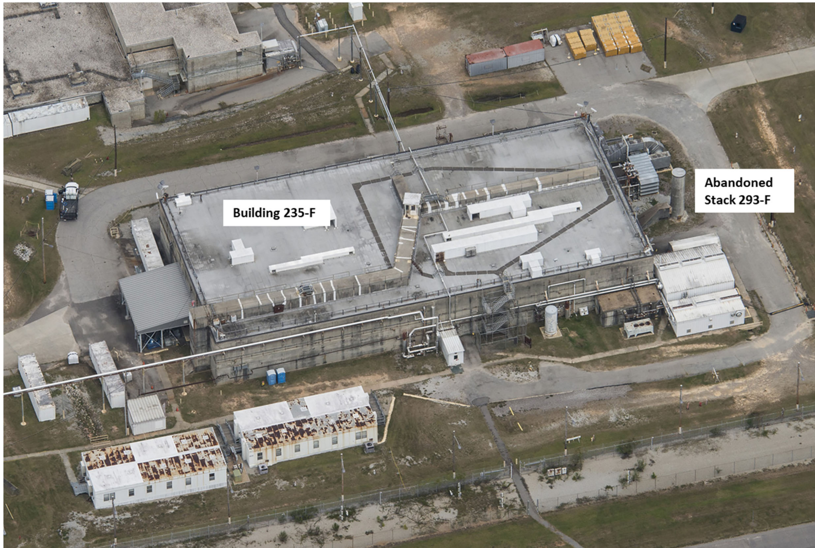
Figure 8. Photograph of Height Reduced Abandoned Capped Stack (293-F)
