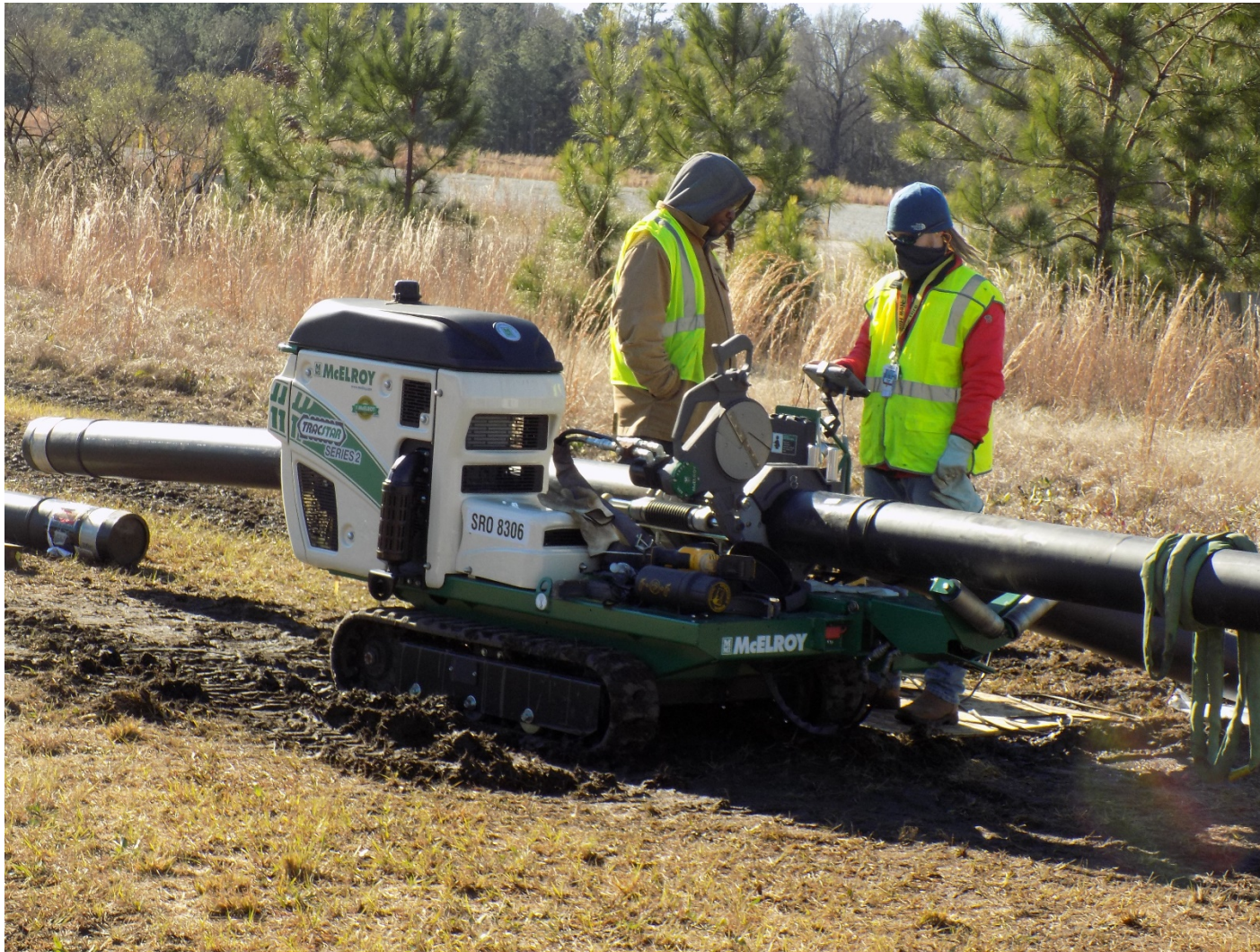
Figure 10. D-Area Treatability Study Pipeline Installation
