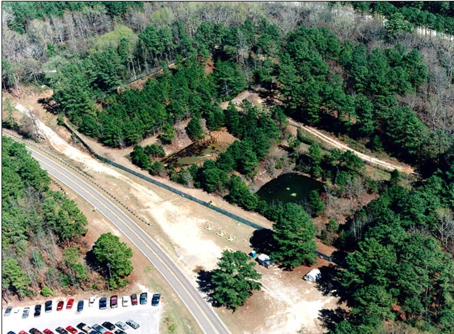
Figure L-3. Photo of SRLSB OU Before Remediation Activities
