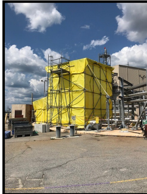
Figure 11: Riser B8 D&R Activities
