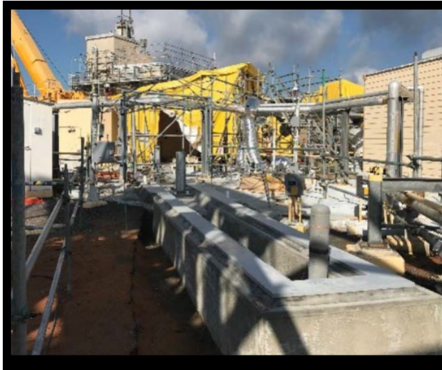
Figure 7: Tank 27F Transfer Line Modifications
