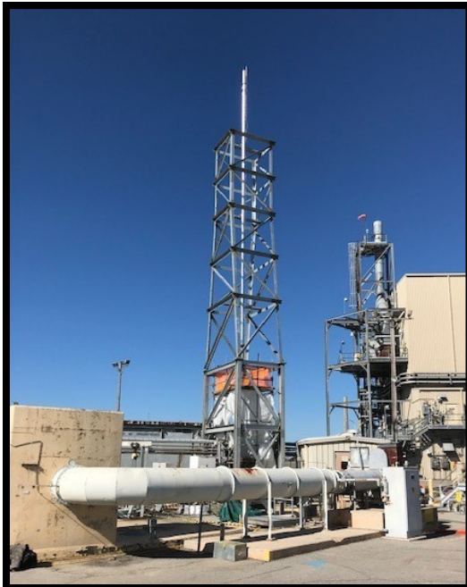
Figure 10: Tank 35H Stack Extension
