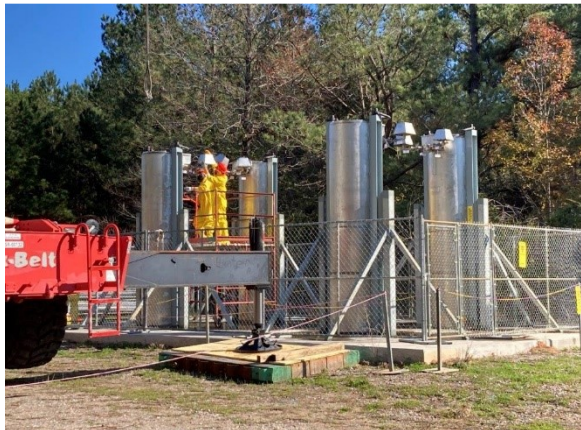
Figure 4: TCCR Columns at ISS Pad
